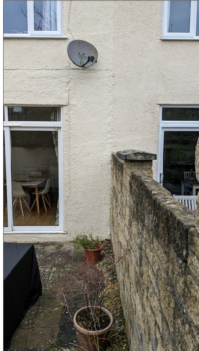
Existing garden Party Wall between host dwelling and attached neighbour (No. 16).
