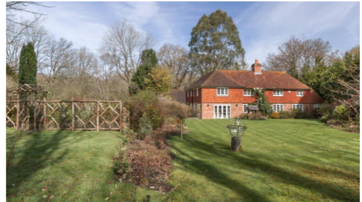
Fig 6 View of Front (South) Facade
