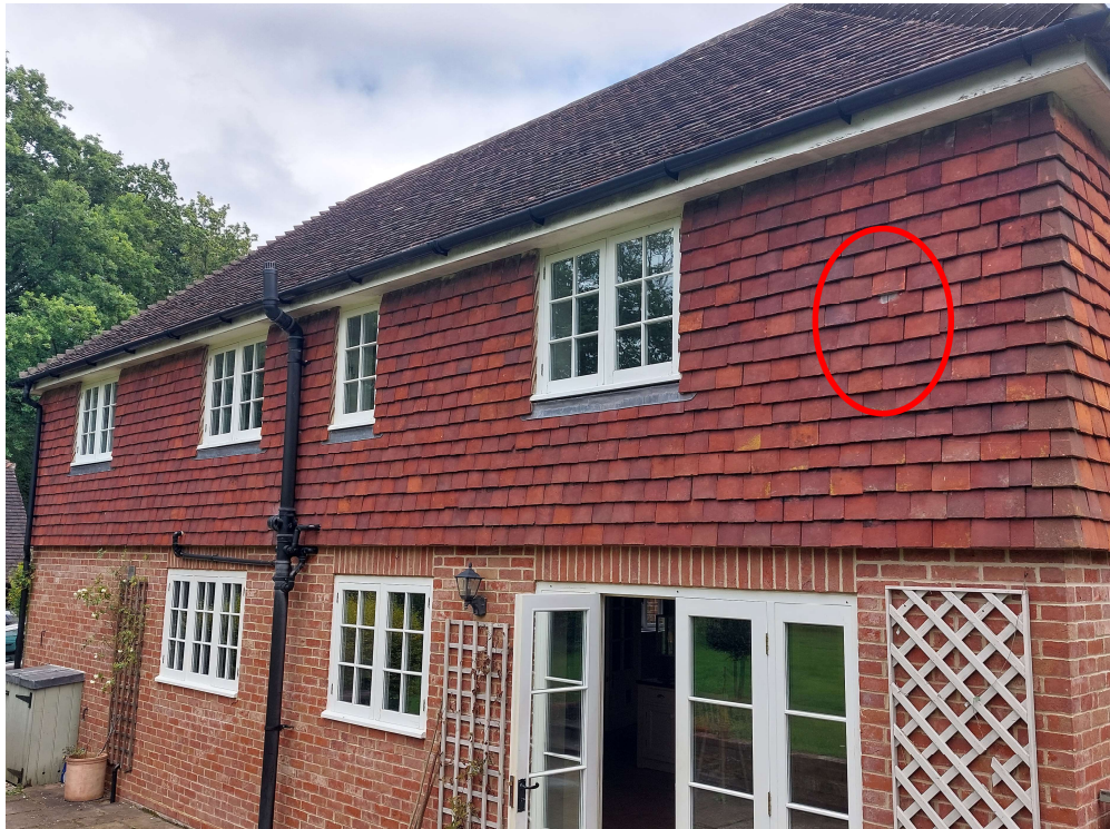
Image No. 01 – B01, western aspect. Pipistrelle access points circled in red.
