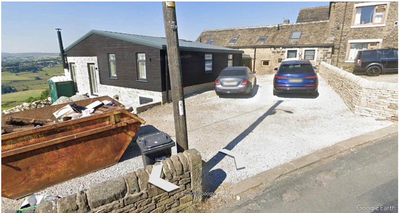
Fig 11: Winterburn Hill Barn conversion to residential showing effective use of shallow sloping metal roof and cladding to retain the impression of farm buildings.
