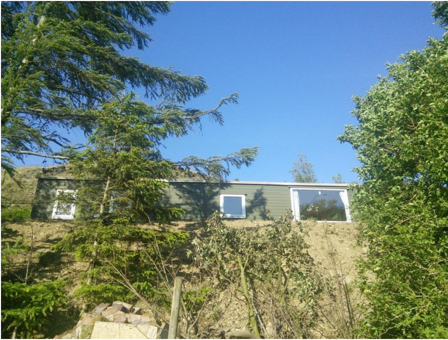
Fig 9: Photograph taken from the bridleway facing east and looking up at about 45 degrees. This was taken in 2017 before the various trees and shrubs grew to their current size. Note that if a sloping roof was added to the top of this building it would not be visible from here on the bridleway.
