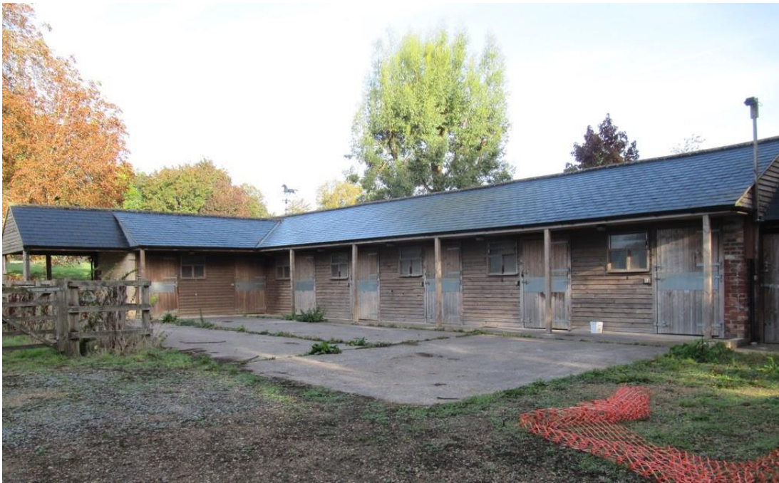
East and south elevations of existing stables
