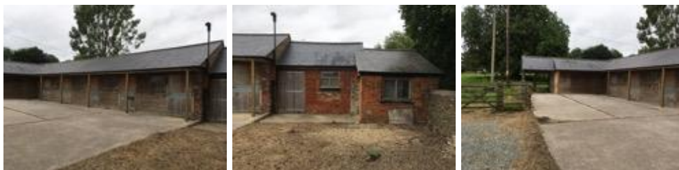
Photographs 1, 2 & 3: External front views of the building
