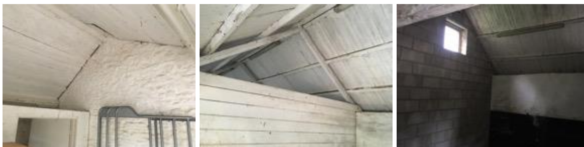
Photographs 5, 6 & 7: Internal views of the main section of the stable
