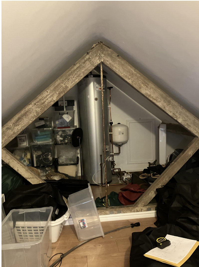
Illustration 2 - Existing roof truss to be retained
