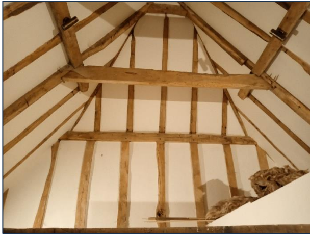
The ceiling voids which show the good quality of the timbers
