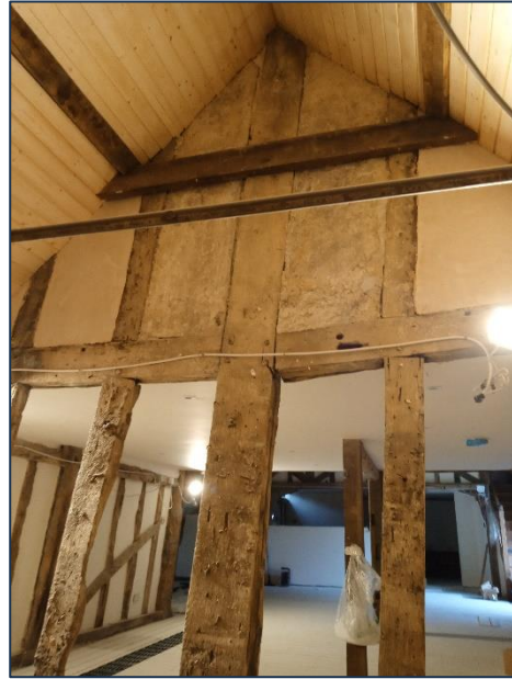
The ceiling voids which show the good quality of the timbers
