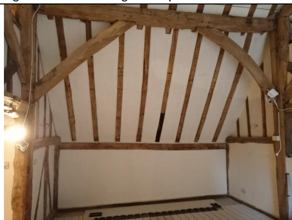
Fig 11. Central bay rear elevation (former porch)
