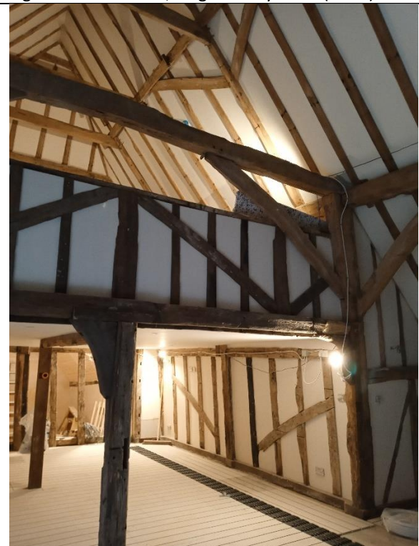
Fig 7. Internal view of South Bays
