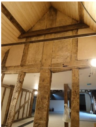
Fig 20. Wattle and daub panels above exposed studs between lean-to and barn
