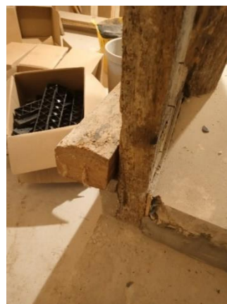
Fig 21. Historically cut soleplate
