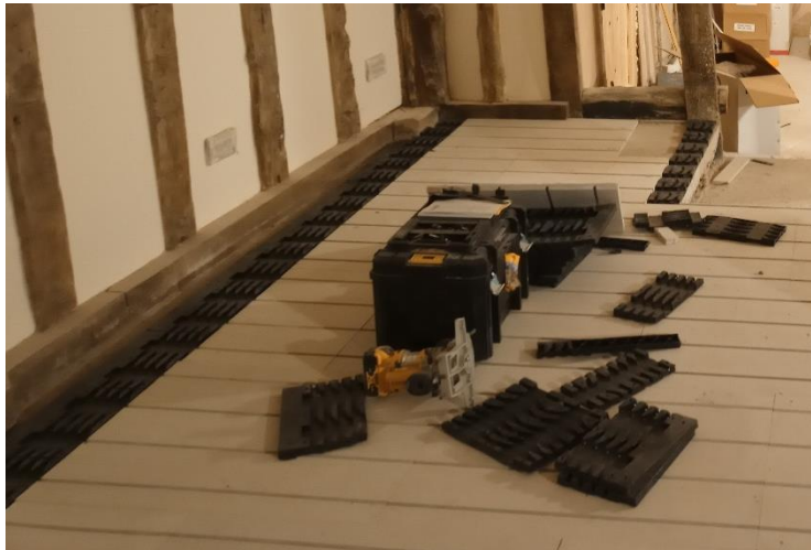
Fig 25. Installation of underfloor heating system over existing concrete slab
