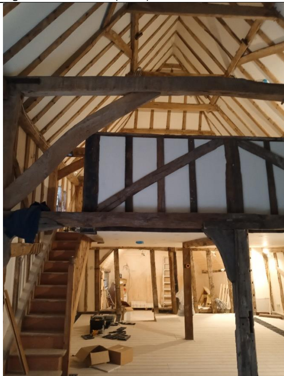
Fig 6. Internal view of South Bays
