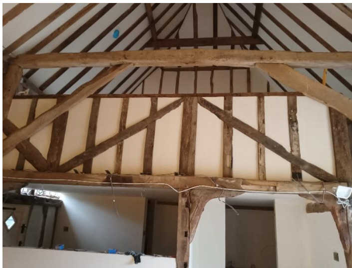
Fig 22. Handrails to mezzanine level
