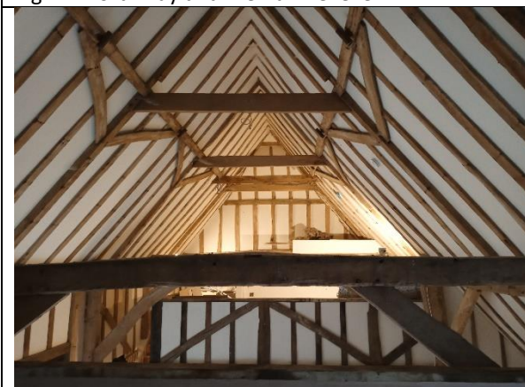
Fig 14. Vaulted ceiling and braces to purlin
