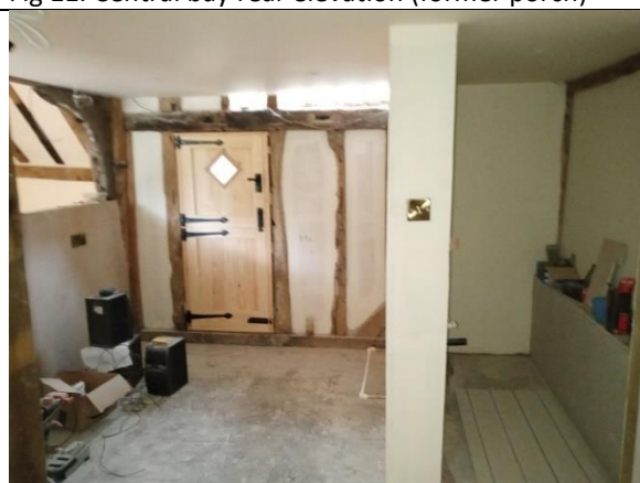
Fig 13. Rear door and stud wall forming WC
