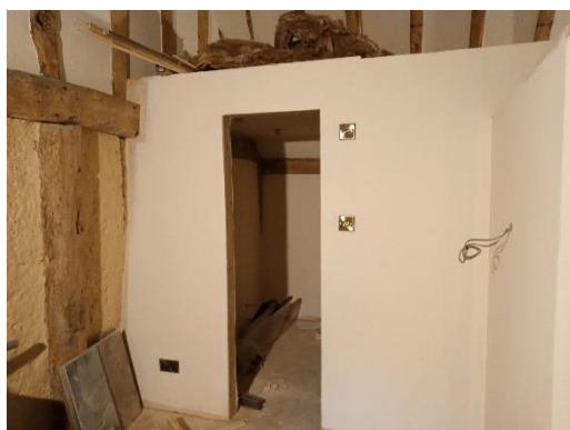
Fig 23. Stud wall to 1 st floor en-suite
