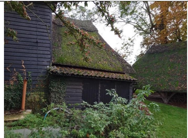
Fig 5. Rear elevation, Single storey store (West)
