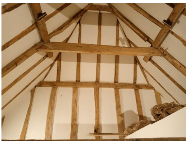
Fig 26. Plasterboard between rafters
