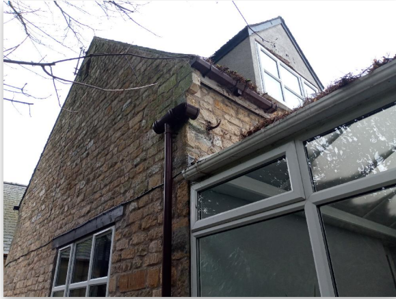
Fig 2.1: No guttering for gully
