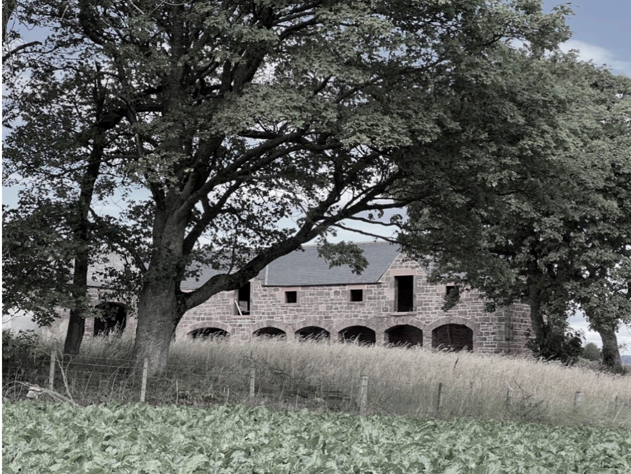
View from SW
