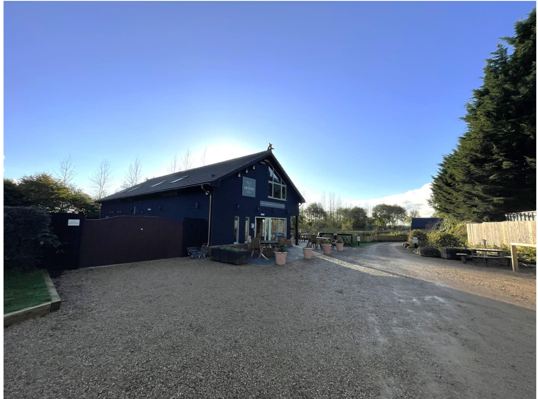
View from the Grange Garden Centre car park – new barrier gate to the Campsite development and 'The Farmhouse' providing visitor amenities
