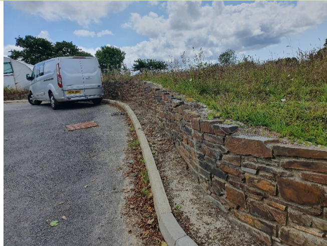
Entrance road comprising of hardstanding
