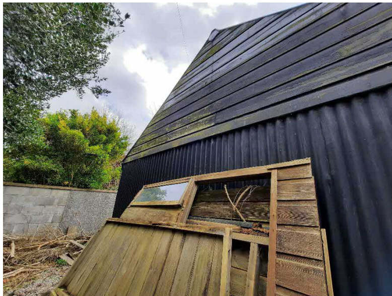
Figure 4: View of the northern elevation of the garage at Carnon Crescent.
