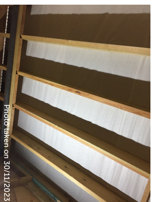
Wooden joists and breathable membrane lined roof of dormer
