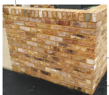
BRICK WALLS TBS London Weathered Brick 1.9m average height
