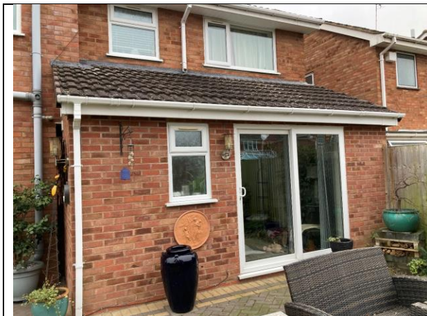
Photo 1 West section sealed
