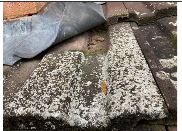
Photo 2 No evidence beneath raised flashing
