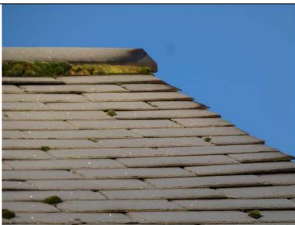
Photograph 5. Further example of the roof slates
