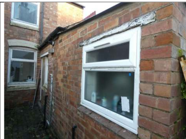
Photograph 11. The sealed south edge of the single-storey rear projection
