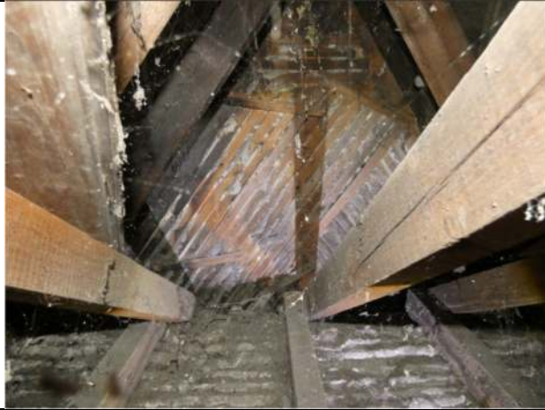
Photograph 14. The area within the roof void in the west dormer gable
