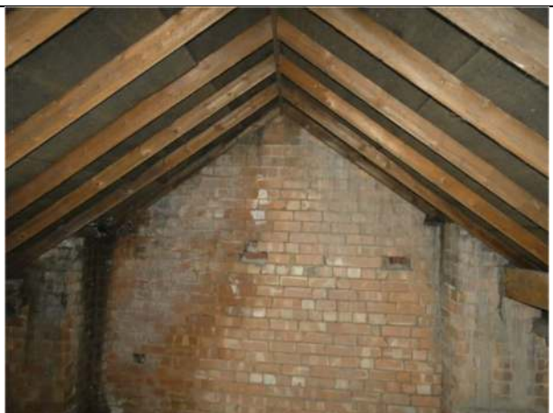
Photograph 12. The enclosed roof void
