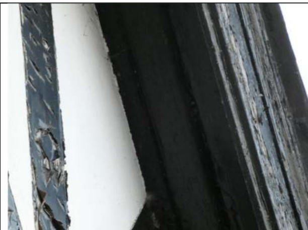
Photograph 9. Example of sealed barge board area on west gable wall
