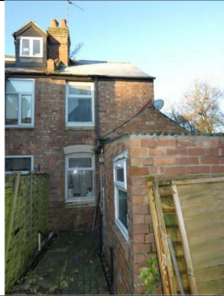
Photograph 2. The east elevation
