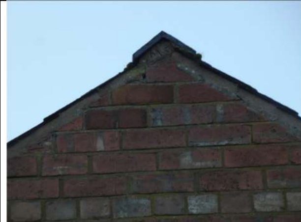
Photograph 7. Example of sealed roof edge on north gable wall
