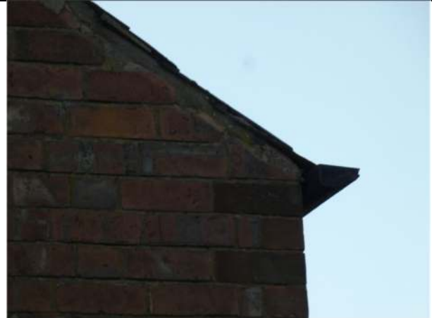
Photograph 8. Further example of sealed roof edge on north gable wall
