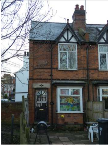
Photograph 1. The west elevation
