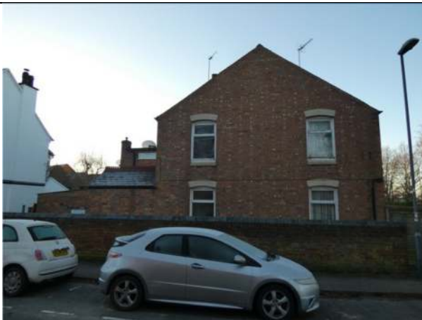
Photograph 3. The north elevation
