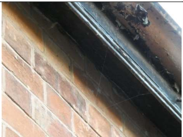
Photograph 10. Example of sealed wooden fascia and soffit
