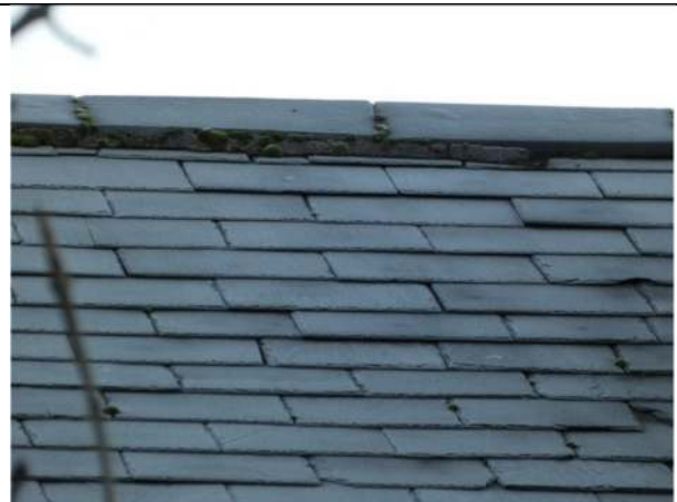
Photograph 4. Example of the roof slates
