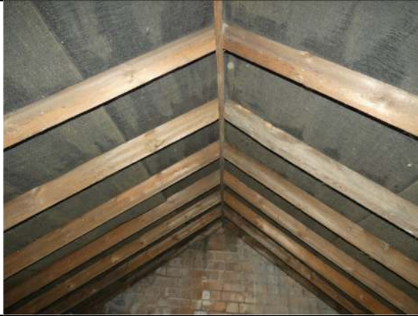
Photograph 13. The ridge area within the enclosed roof void
