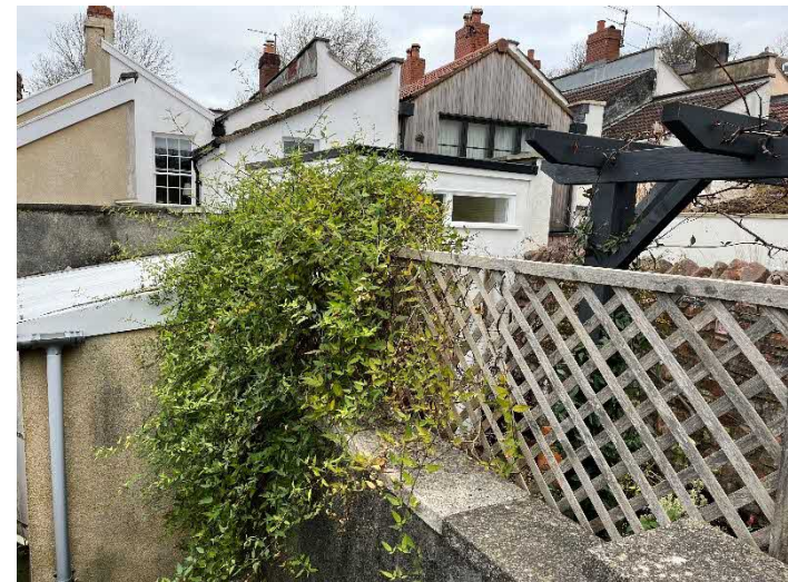
Photo 12. The rear of the property, northern boundary wall shared with no. and view towards the infill extension built at the rear of no. 4 Church Lane (PP ref. 18/04726/H).
