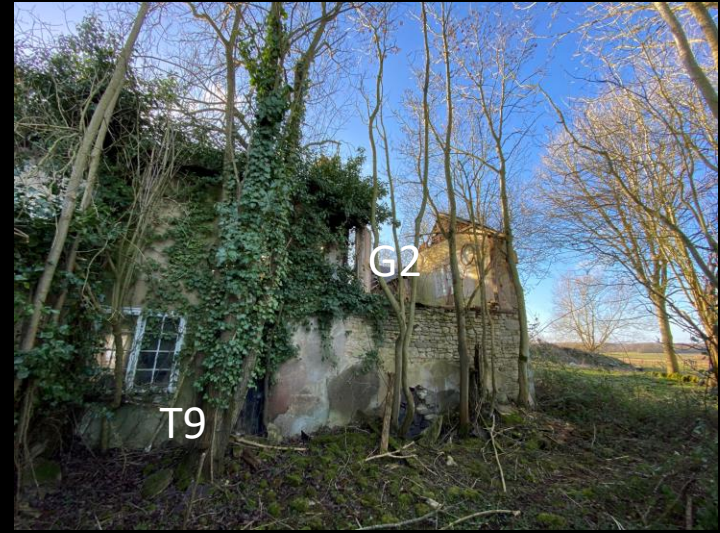
Typical cover around building, north side
