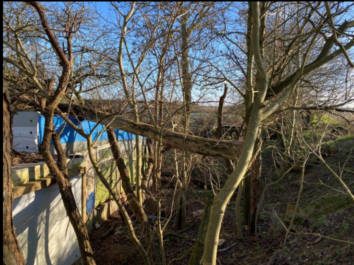
Collapsed tree over container – G5
