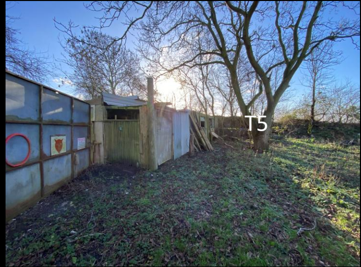
Container and lean-to forming 'barn' area near T5
