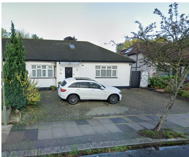
Overall view of the property from High View Gardens
