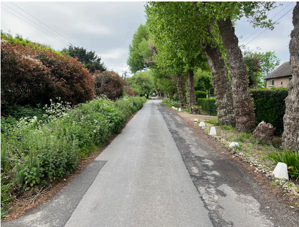
Chalk Lane looking south towards the site access on LHS
