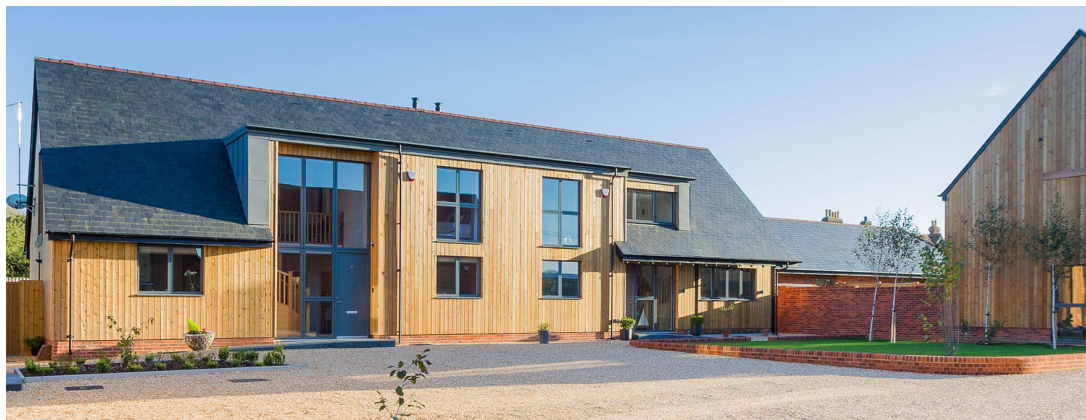
Example of semi rural development utilising rustic rough sawn timber over brick plinth: Buckland Granaries
