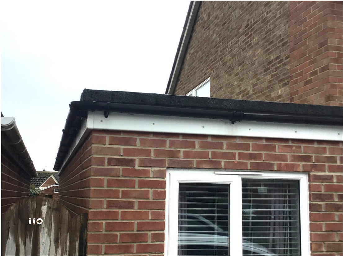
Figure 3. Side extension west and north elevations looking east.
