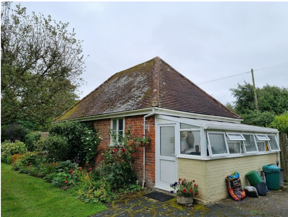
Photo 4 – West facing elevation.
