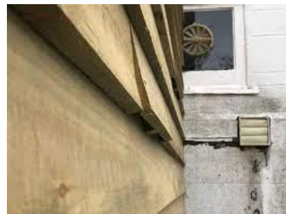
Figure 9 – Pegged cladding technique
