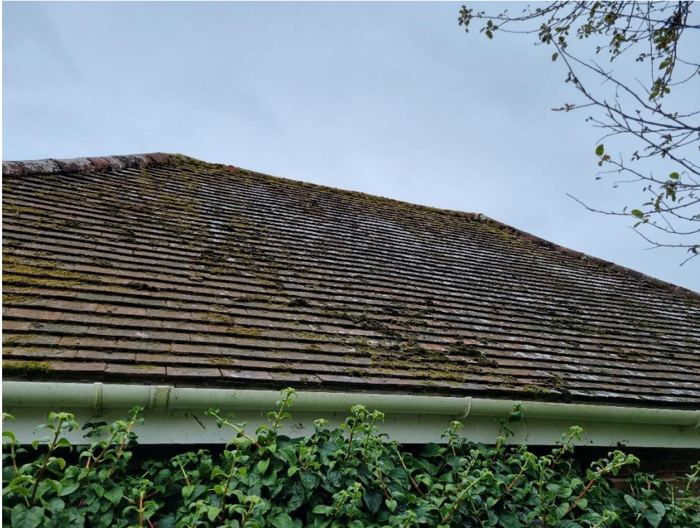
Photo 3 – West facing roof.
