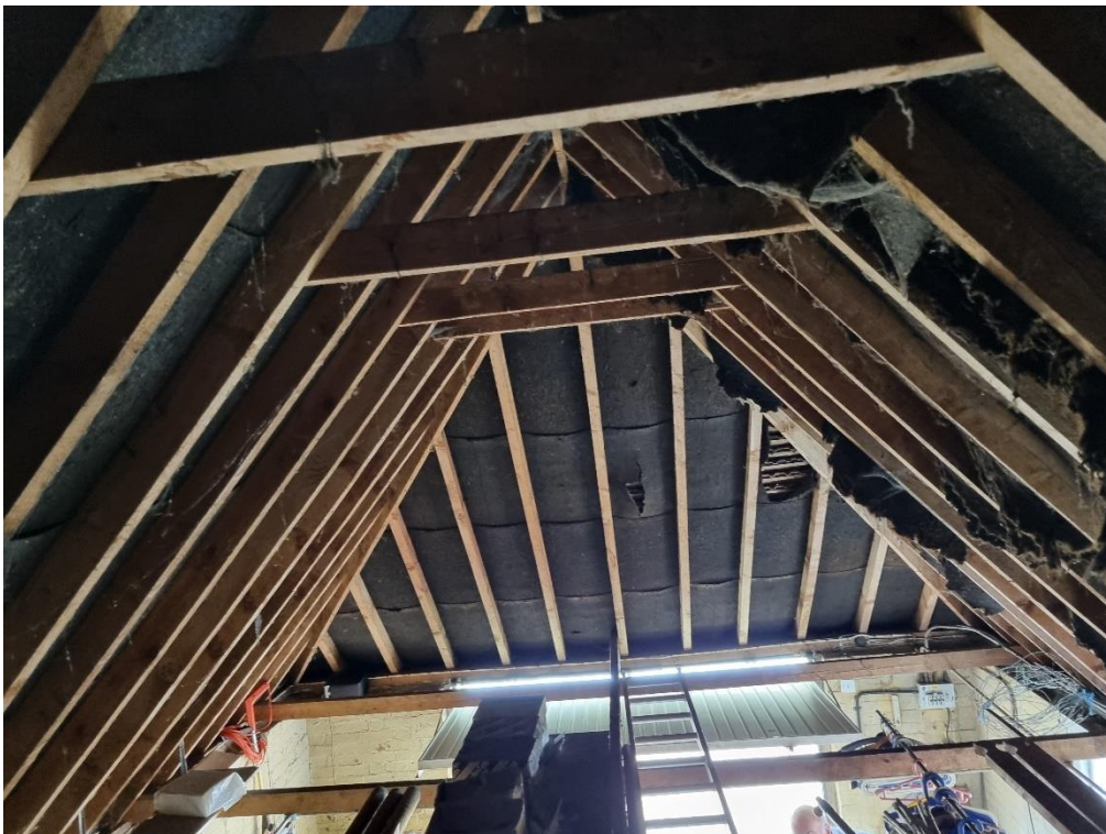
Photo 6 – Interior loft and roof space.
