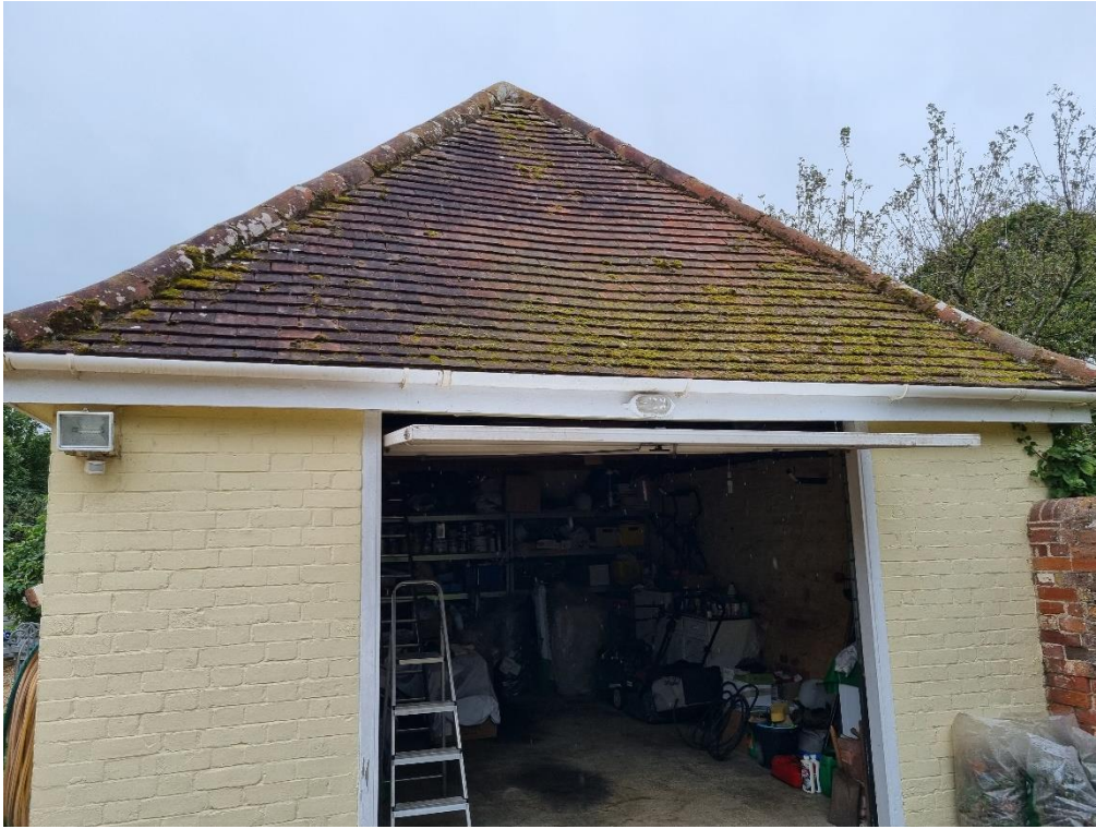
Photo 1 – North facing elevation.
