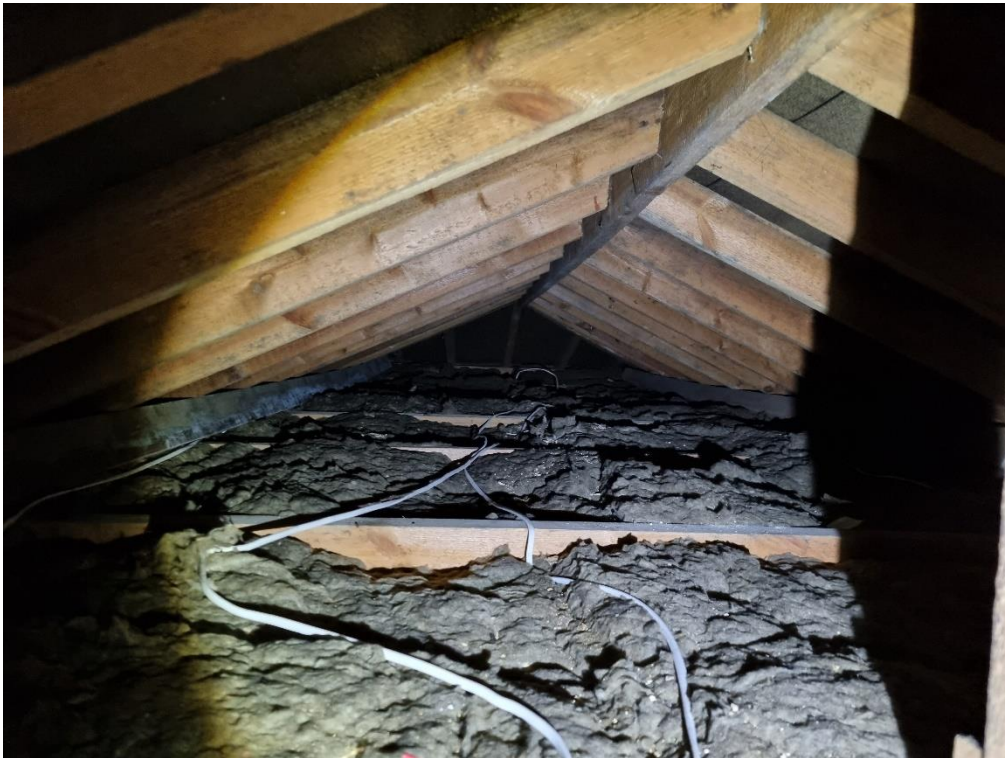
Photo 8 – Interior loft void.
