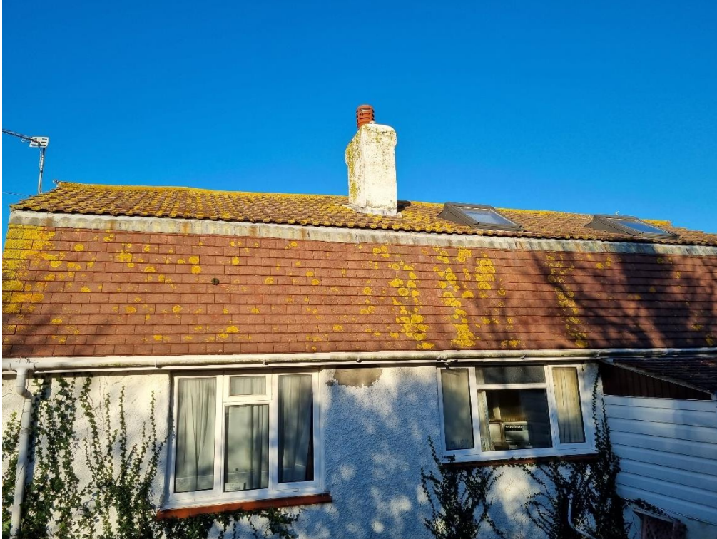
Photo 5 – South elevation roof tiles.
