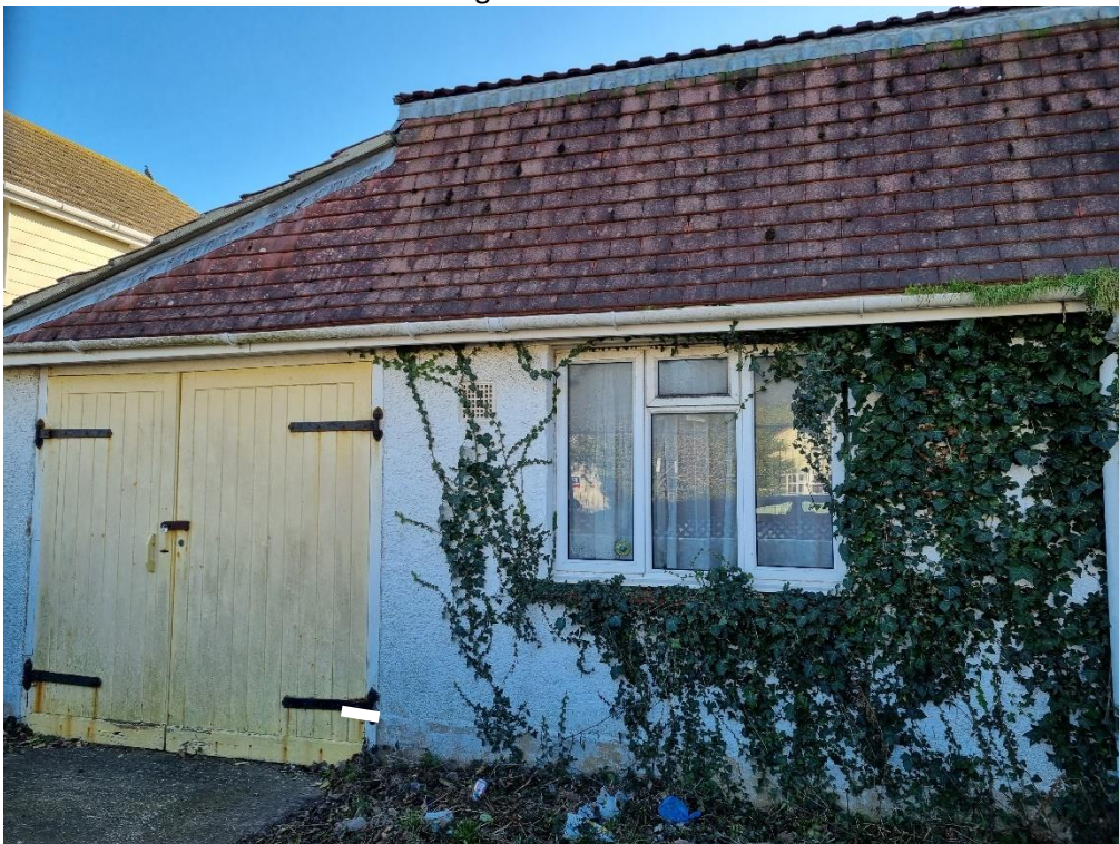
Photo 4 – Garage doors on north elevation.
