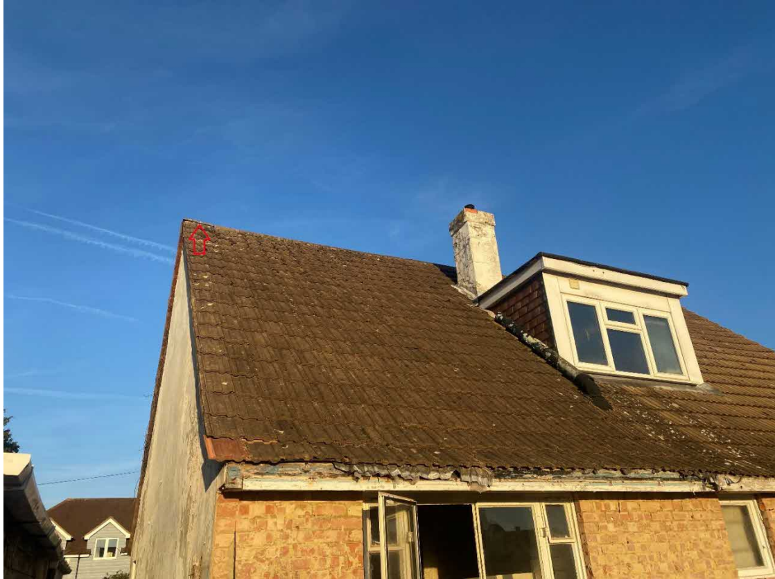
Figure 1. North and west elevation looking east.
