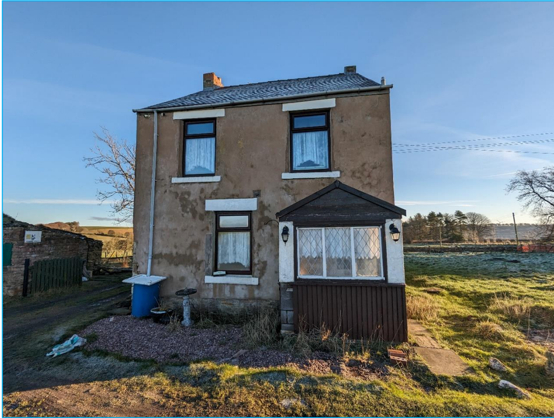
Photograph 8 – West elevation with single-storey, pitched roof extension.
