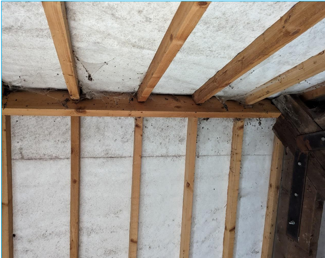
Photograph 11 – Breathable slate roof lining and cobwebs in roof void.
