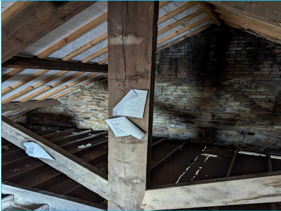
Photograph 10 – King post roof void and inside of south gable.
