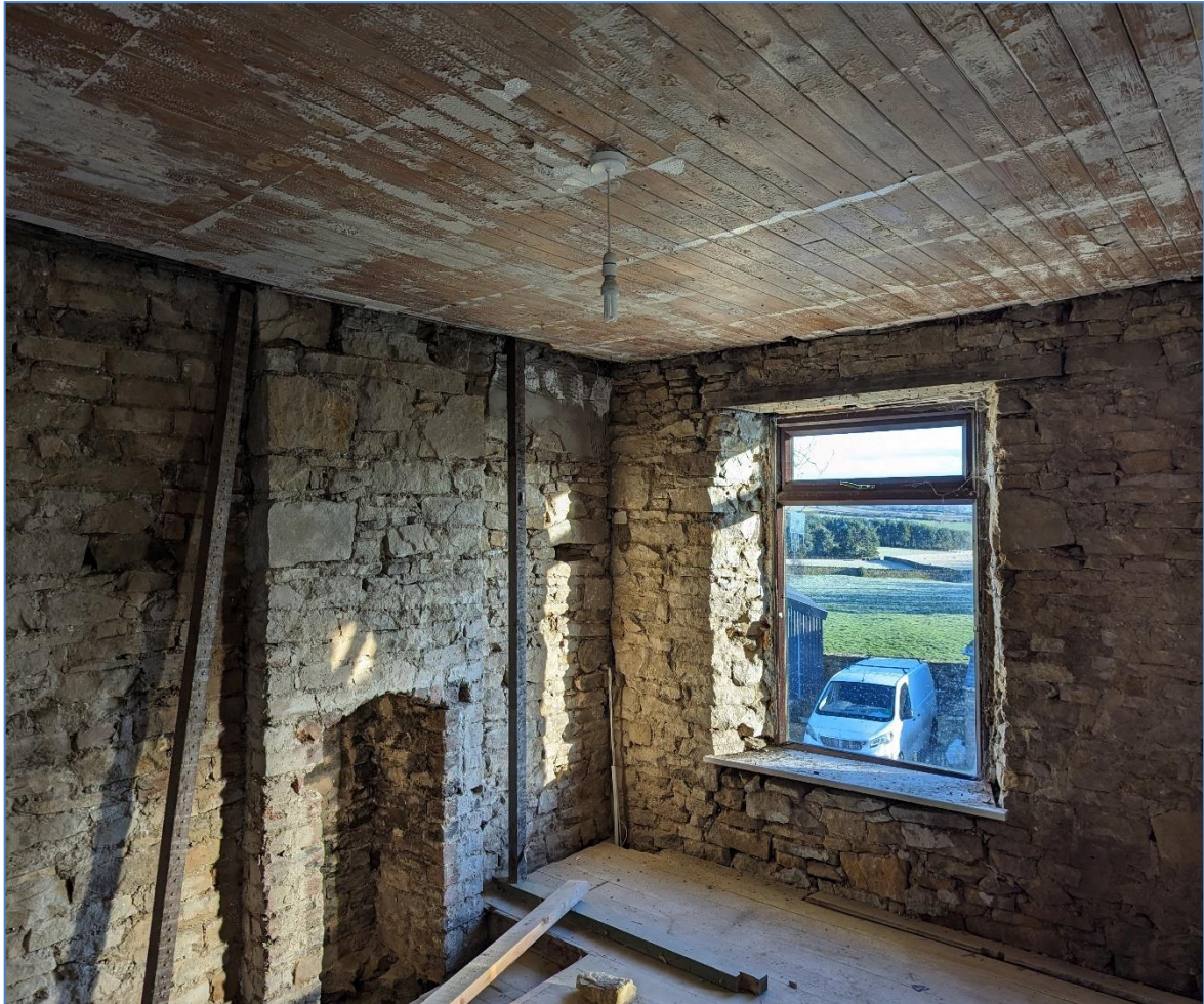
Photograph 1 – Soft stripping and dismantling inside Lark House.
