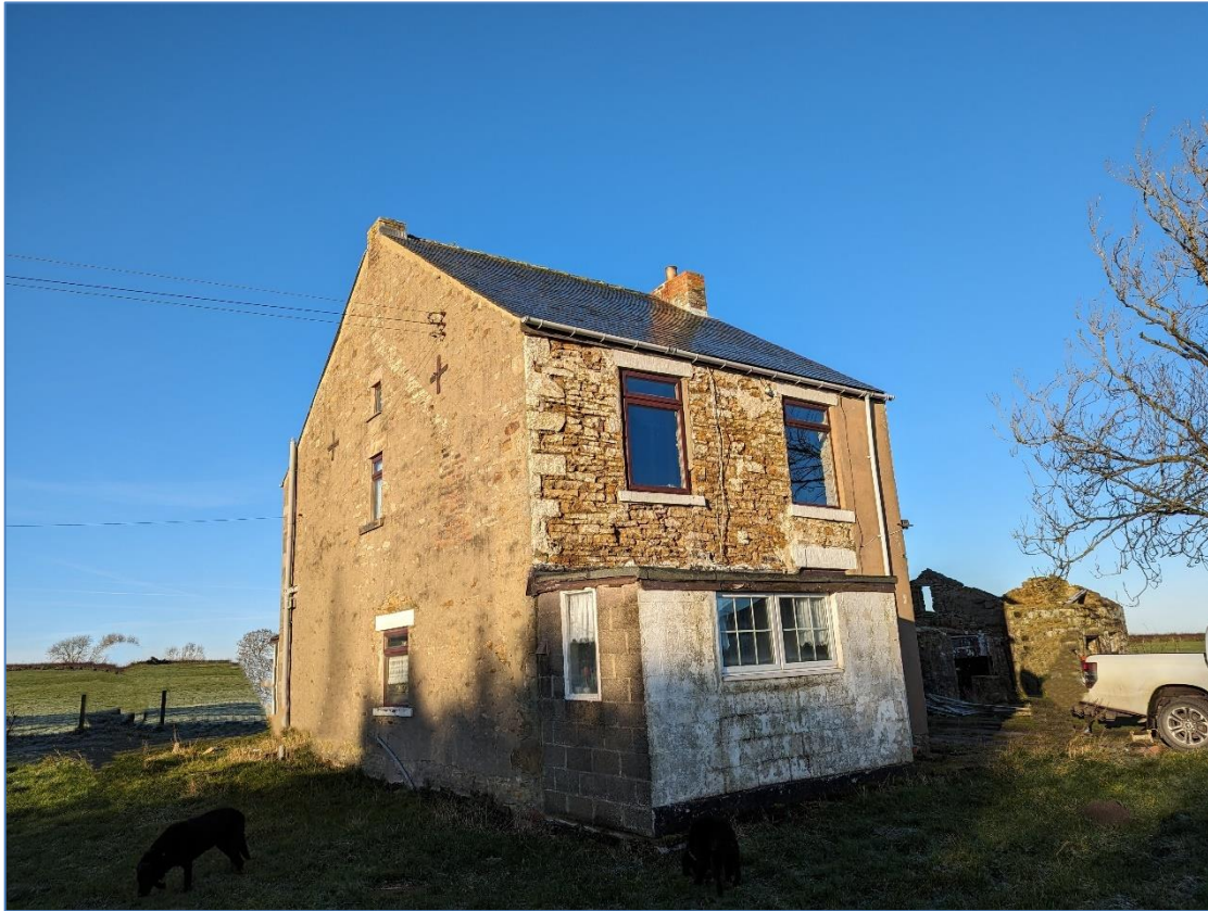
Photograph 2 – Pitched slate roof and lead flashing round chimney bases.
