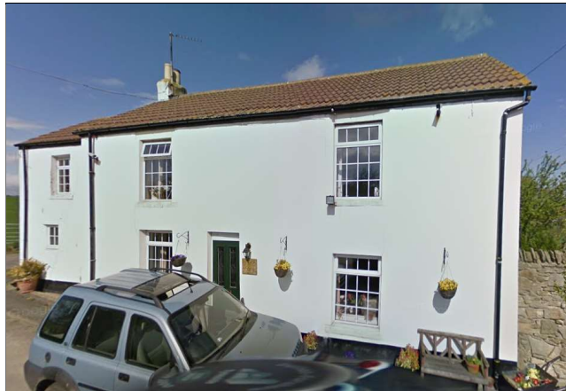
Photograph 4 – Adjacent Lark Cottage with clay pan tile roof covering
