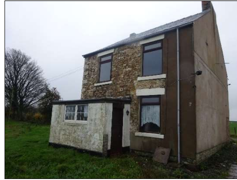
Photograph 3 – East view of main building
