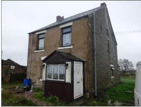
Photograph 2 – West view of main building
