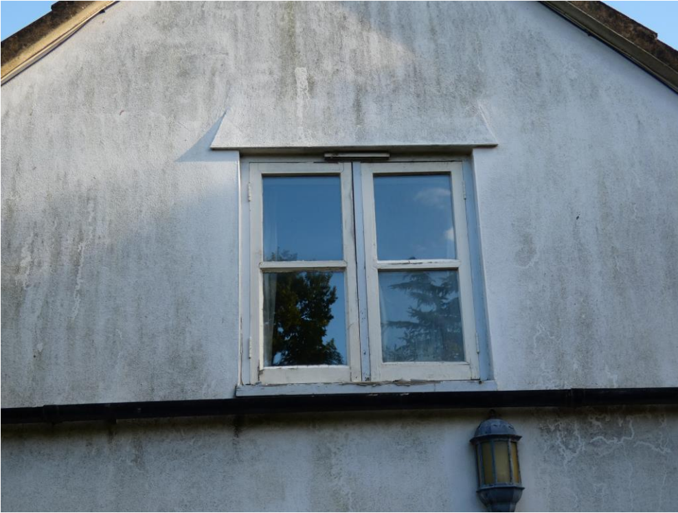
Rear FF Lefthand window (F) (to be replaced as existing)
