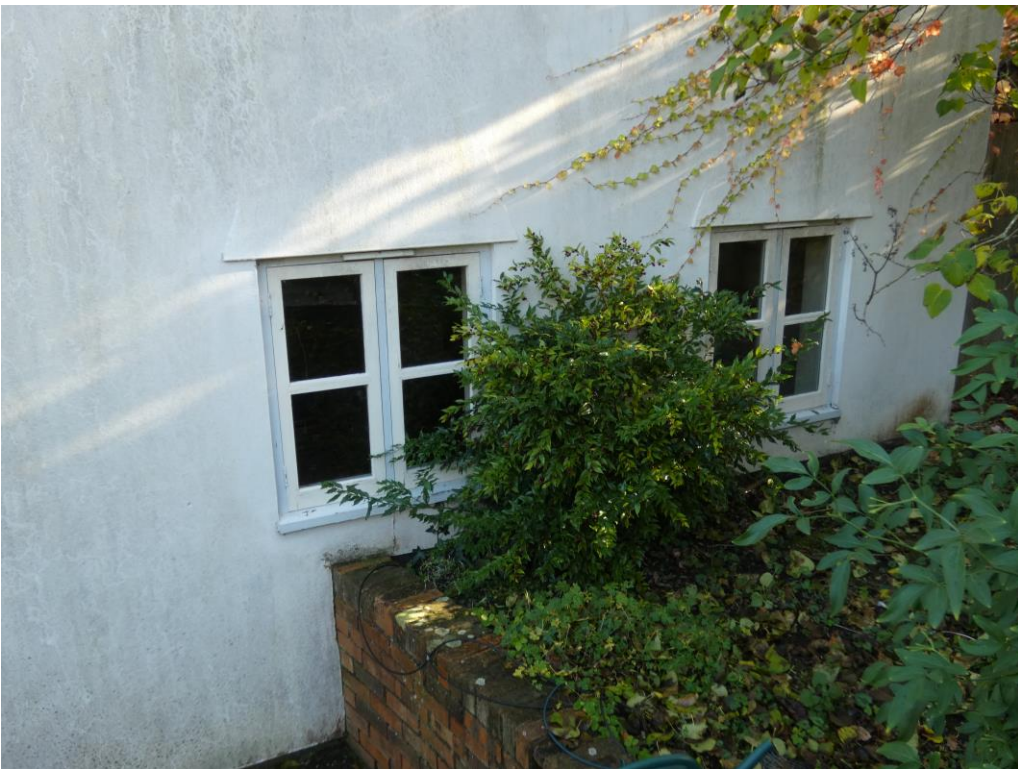
Rear GF Righthand windows (H)(I)(to be replaced with glass doors)
