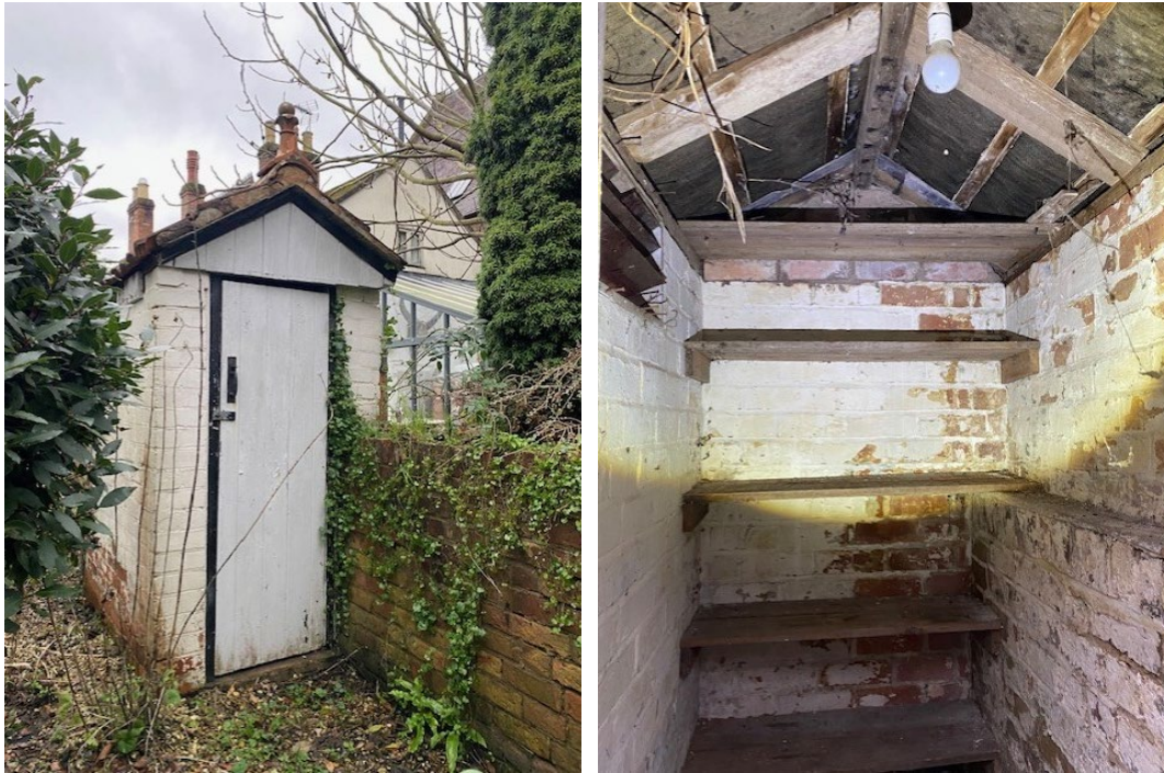
Small outbuilding to the south-east of the house
