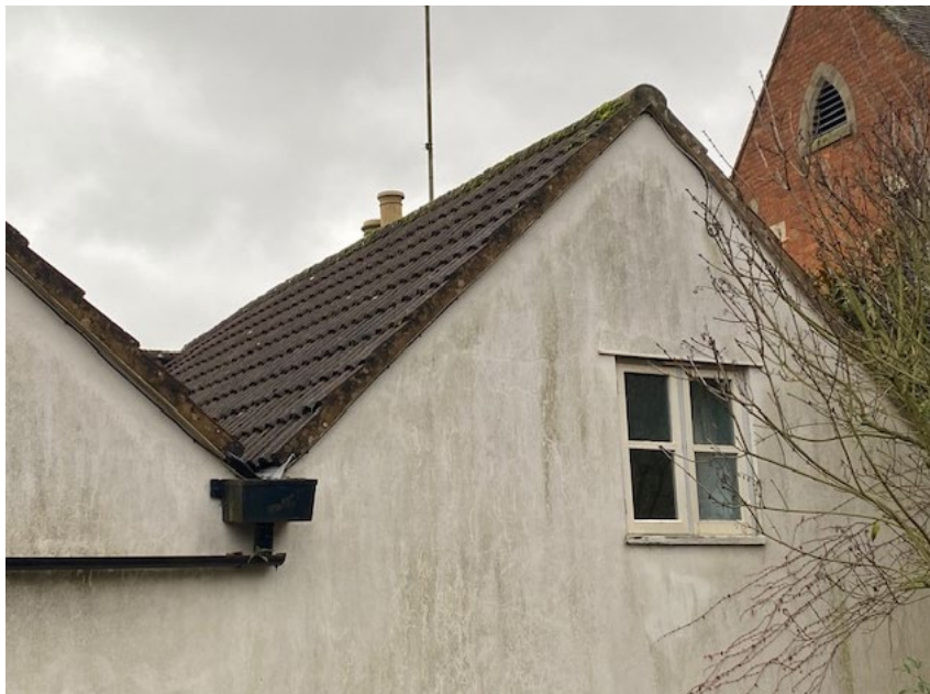
South gable roof section, south side slope and gable end
