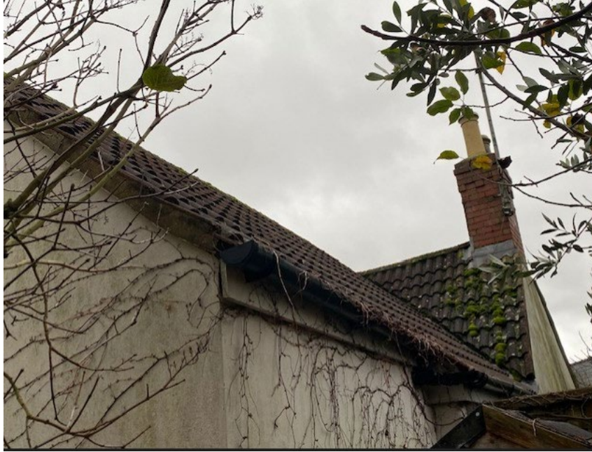
South gable roof section, north side slope
