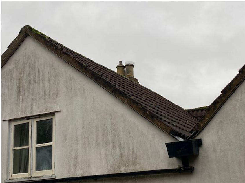
North gable roof section, south side slope and gable end
