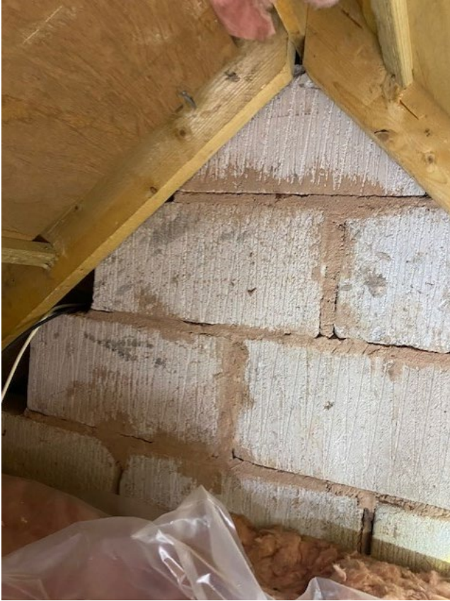
Internal view of west gable wall inside southern rear loft
