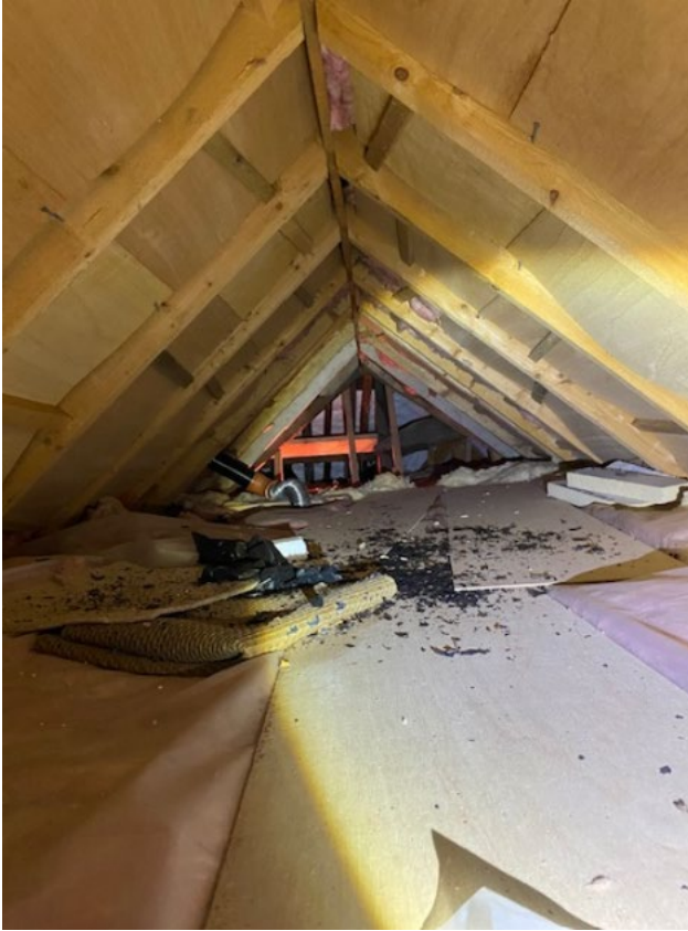
Northern rear loft void
