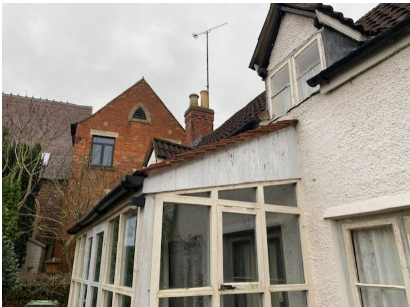
End tiles are well bedded in on side of porch
