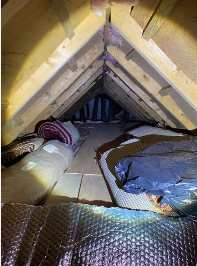
Southern rear loft void
