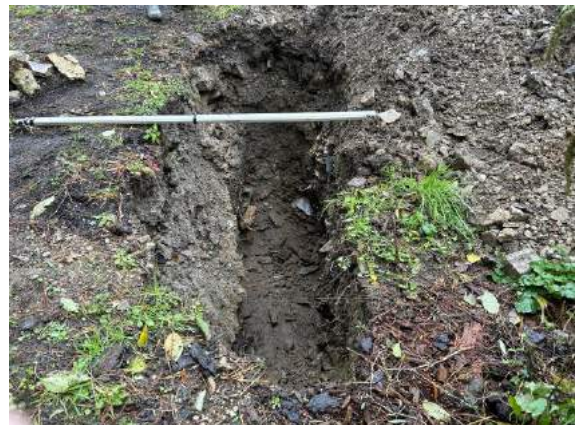
Photo 11: TP01 Test 3 completed (12 mins) from Face B looking 095 E
