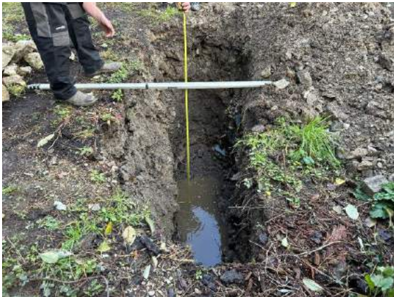
Photo 9: TP01 Test 2 in-progress (4 mins 30 secs) from Face B looking 095 E
