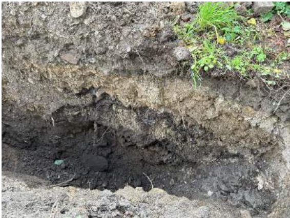
Photo 3: Completed TP01 from Face C looking 185 S
