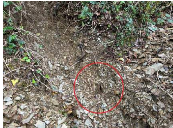
Photo 14: Prior cut to the east showing underlying weathered Bedrock over Bedrock
