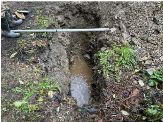
Photo 10: TP01 Test 3 in-progress (3 mins) from Face B looking 095 E
