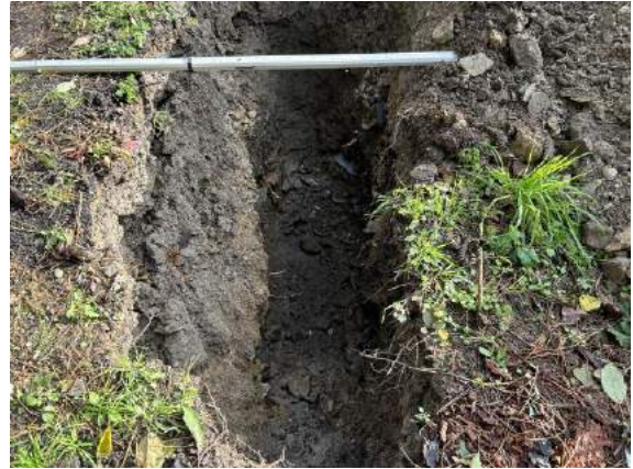
Photo 8: TP01 Test 1 completed (8 mins 15 secs) from Face B looking 095 E
