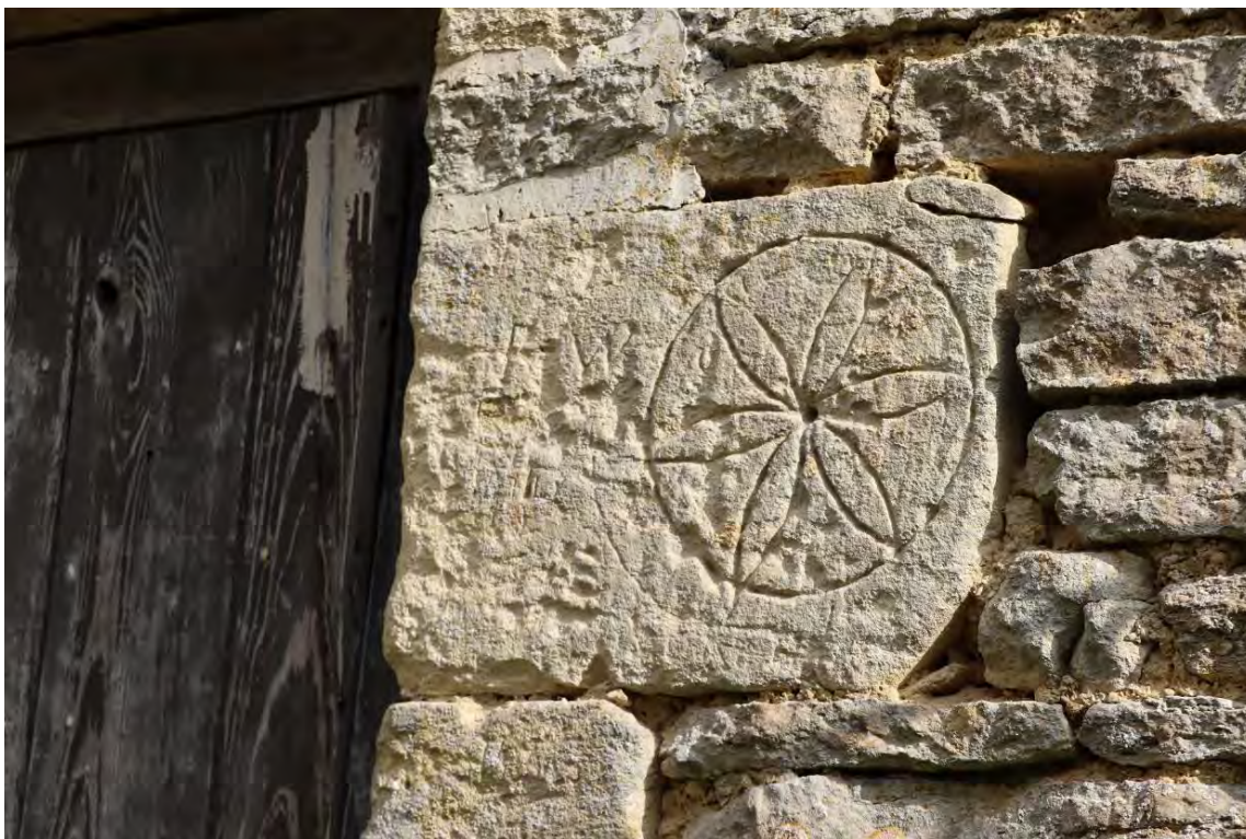
Plate 53: Detail of 'daisy wheel' apotropaic mark on quoin to south elevation of threshing porch, Barn 1 (West)
