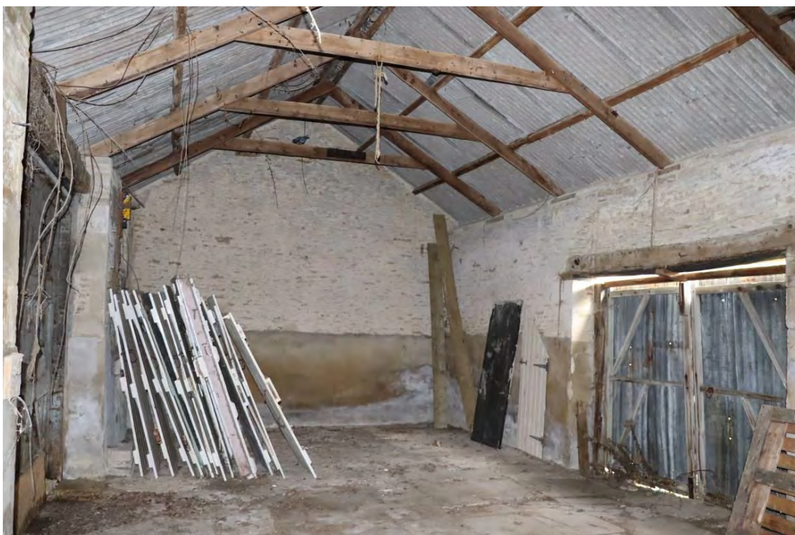
Plate 62: Barn 1 (East), looking east
