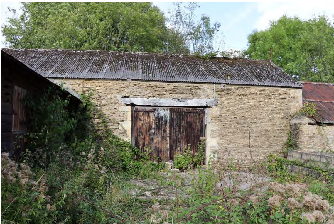
Plate 61: Barn 1 (East), front elevation
