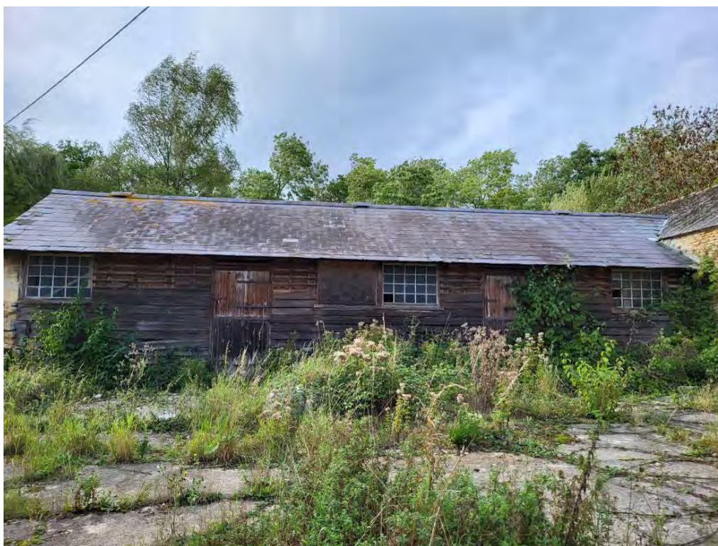
Plate 80: Barn 5: east elevation
