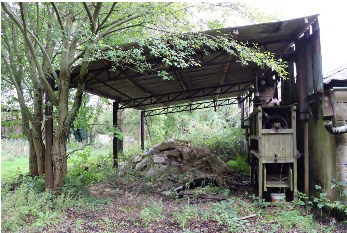
Plate 65: Later 20 th -century steel-framed structure attached to rear elevation of Barn 2, looking east
