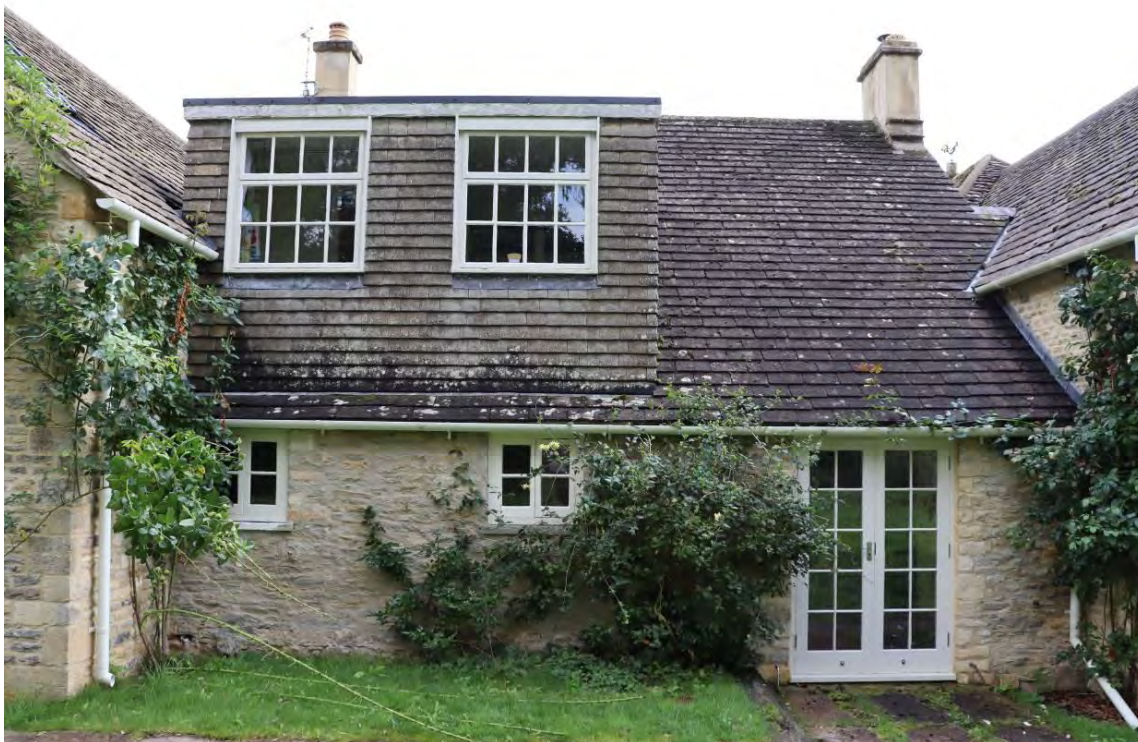
Plate 6: Detail of rear elevation of central range
