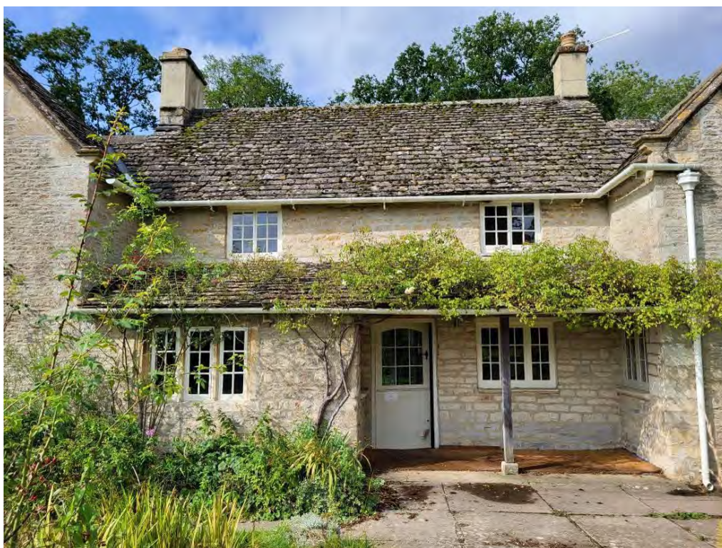
Plate 3: Front elevation: detail of central range
