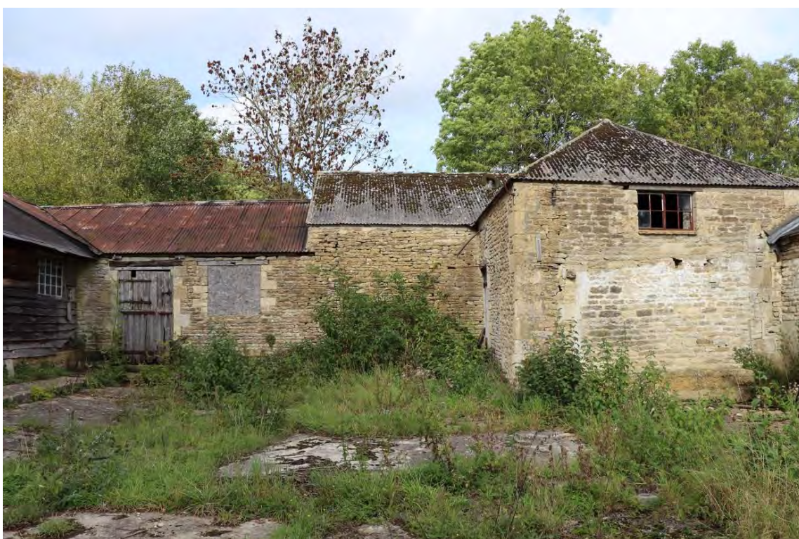
Plate 50: Barn 1 (West) with infilled threshing porch to right and Barn 2 to left
