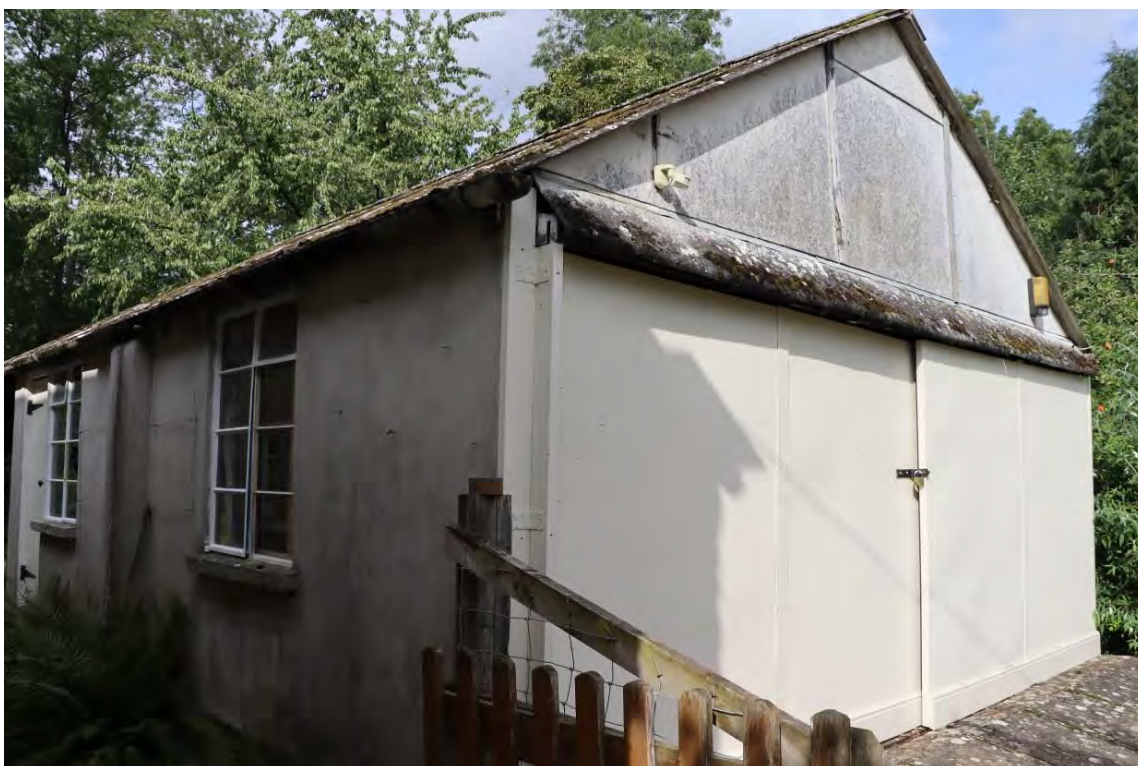
Plate 9: 1960s' garage building
