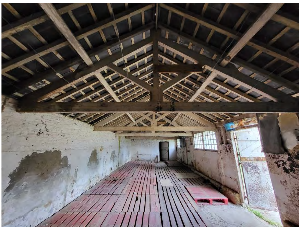
Plate 72: Barn 3, looking north
