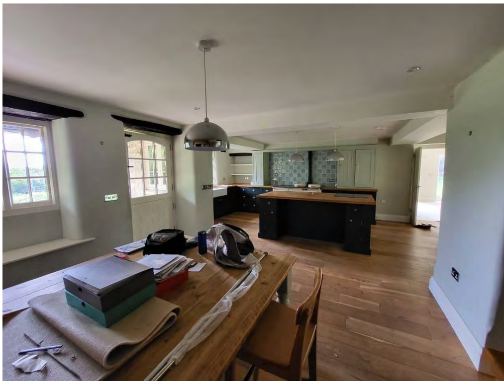
Plate 13: G1, looking south through cut-away wall into G2
