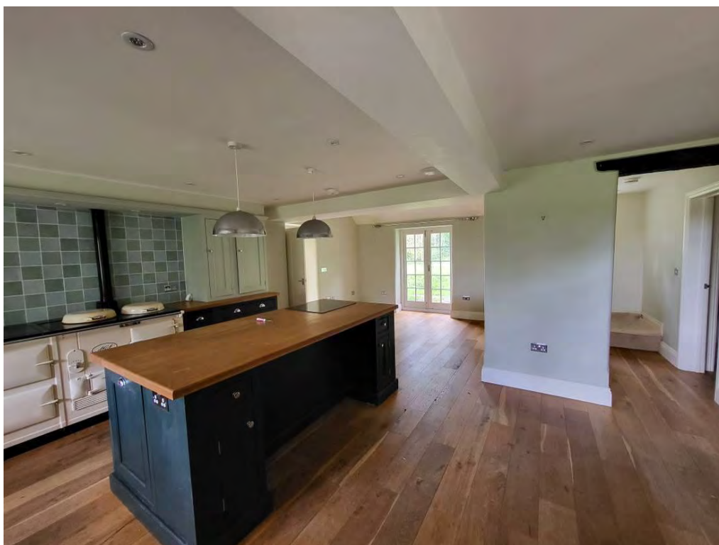
Plate 14: G2, looking west into G3 through cut-away wall
