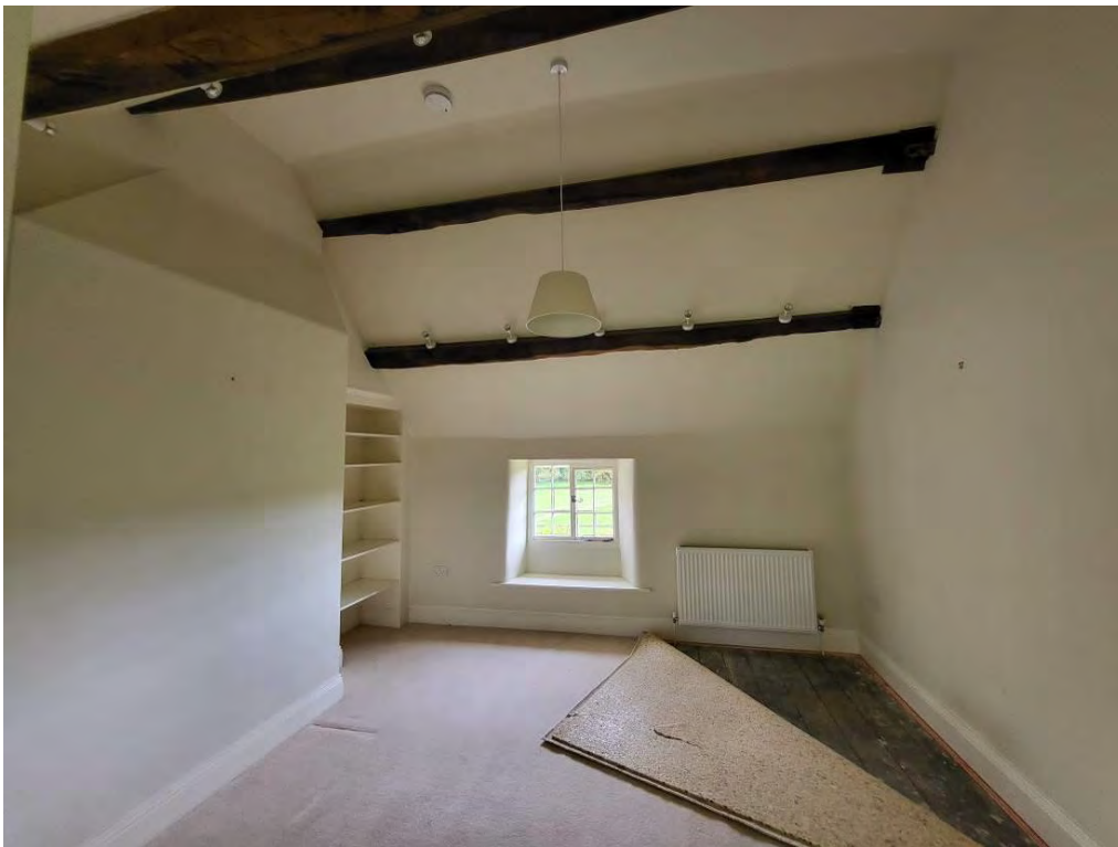
Plate 31: F3, looking east
