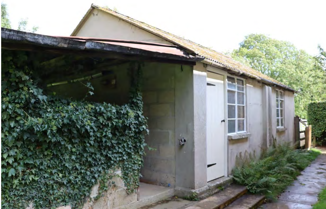
Plate 10: 1960s' garage building
