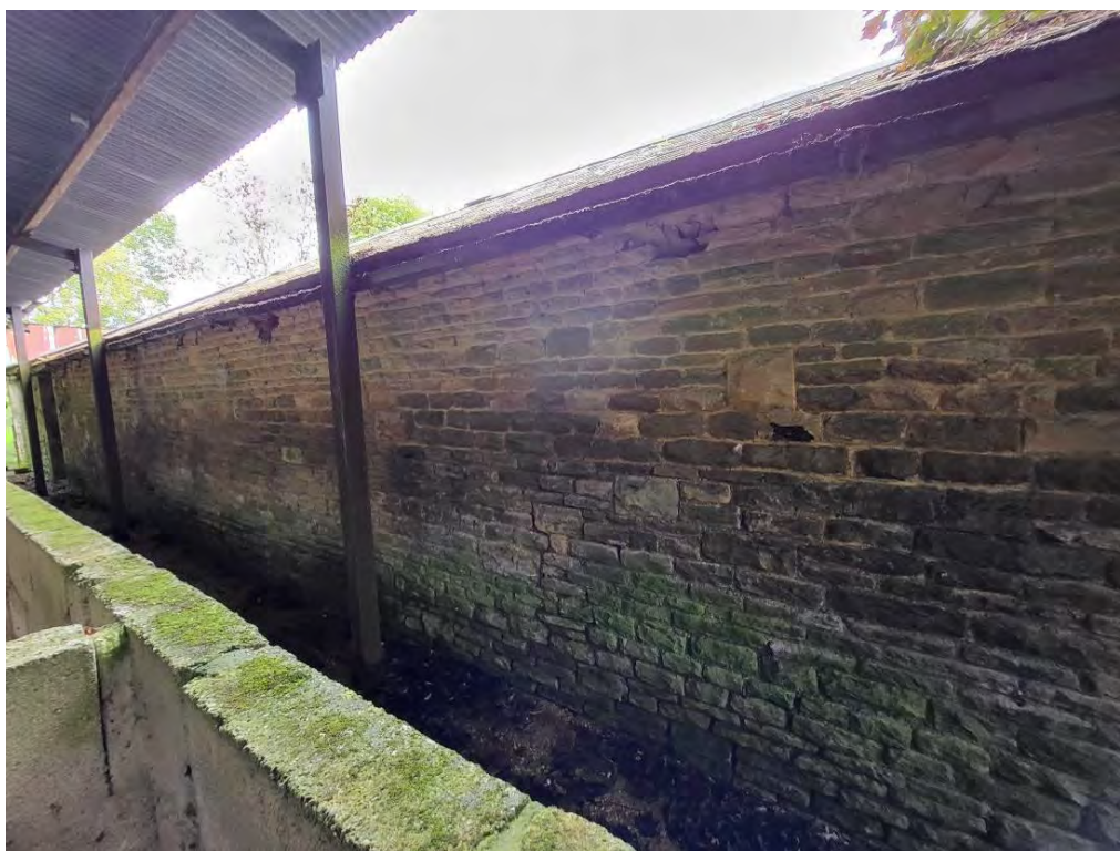
Plate 70: Barn 3, rear elevation, with steel frame of adjoining Barn 6
