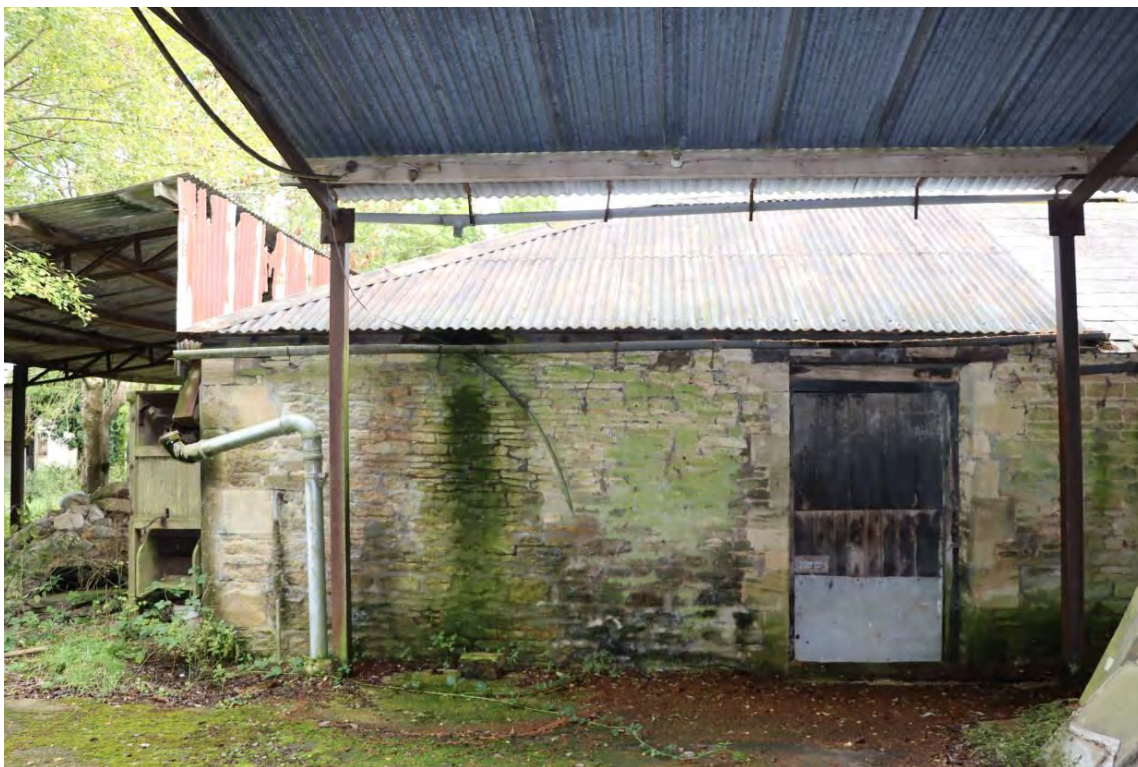
Plate 71: Barn 3, rear elevation, with steel frame of adjoining Barn 6
