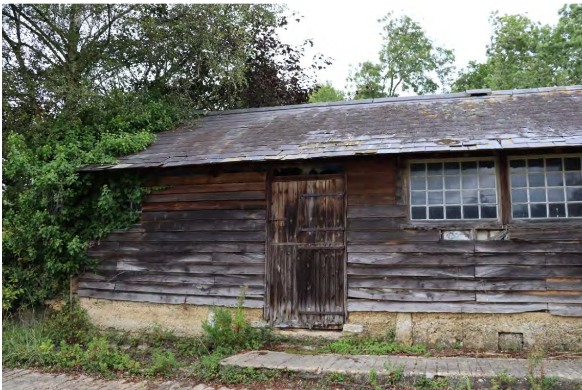
Plate 69: Barn 3, front elevation, note staddle-stones in plinth
