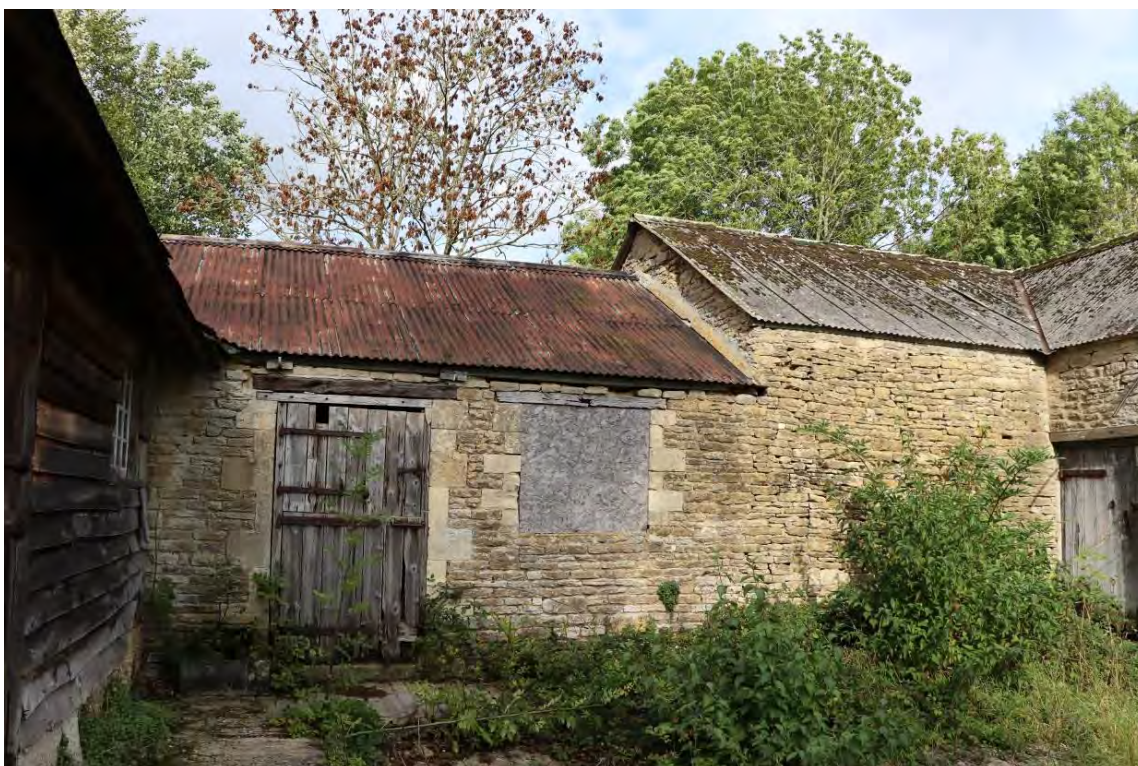
Plate 64: Barn 2, front elevation
