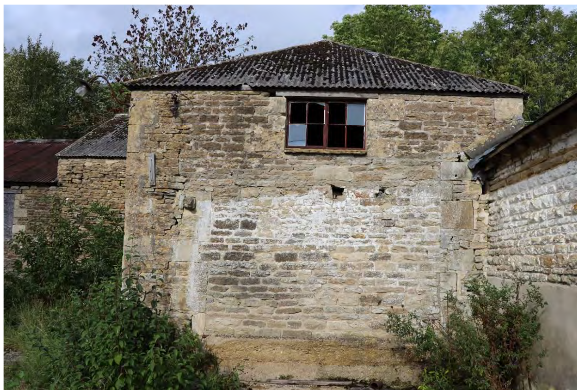
Plate 52: Detail of threshing porch to Barn 1 (West), with infilled opening
