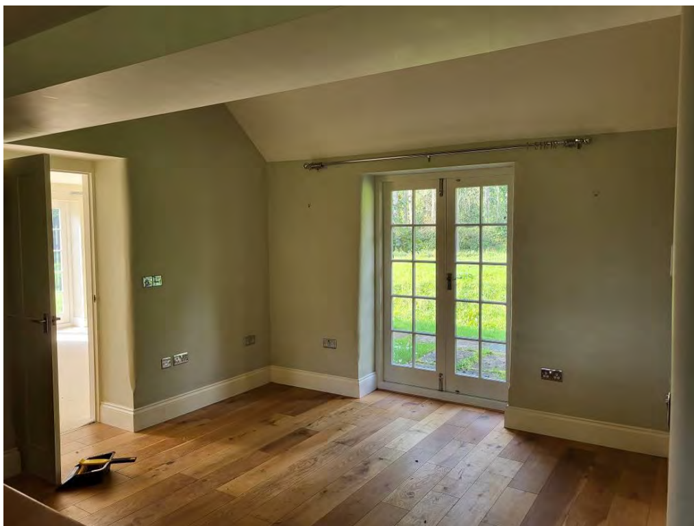
Plate 16: G3, looking west, with door into 2013 extension to left
