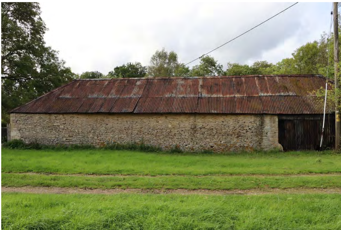
Plate 77: Barn 4: east elevation
