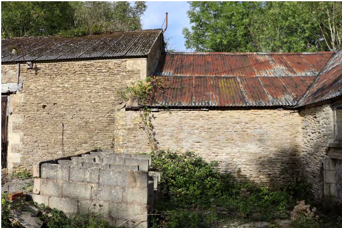
Plate 74: Barn 4: southern elevation to courtyard
