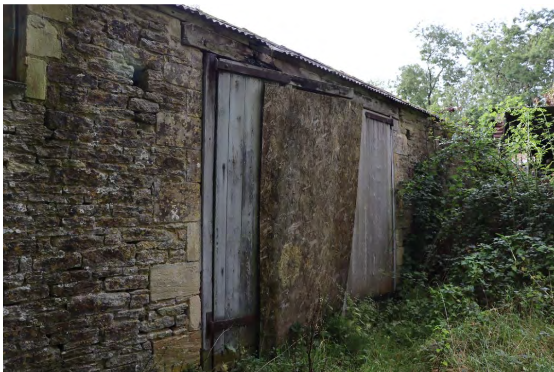
Plate 55: Threshing bay entrance in rear elevation of Barn 1 (West)
