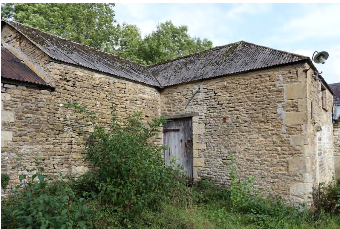
Plate 51: Barn 1 (West), detail of west elevation of threshing porch)
