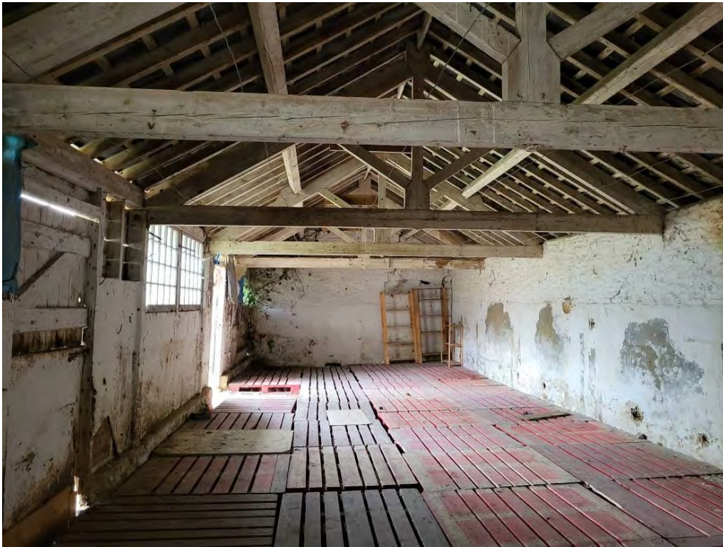
Plate 73: Barn 3, looking south
