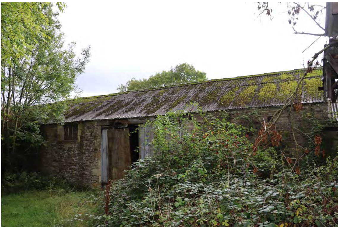
Plate 54: Rear elevation of Barn 1 (West)
