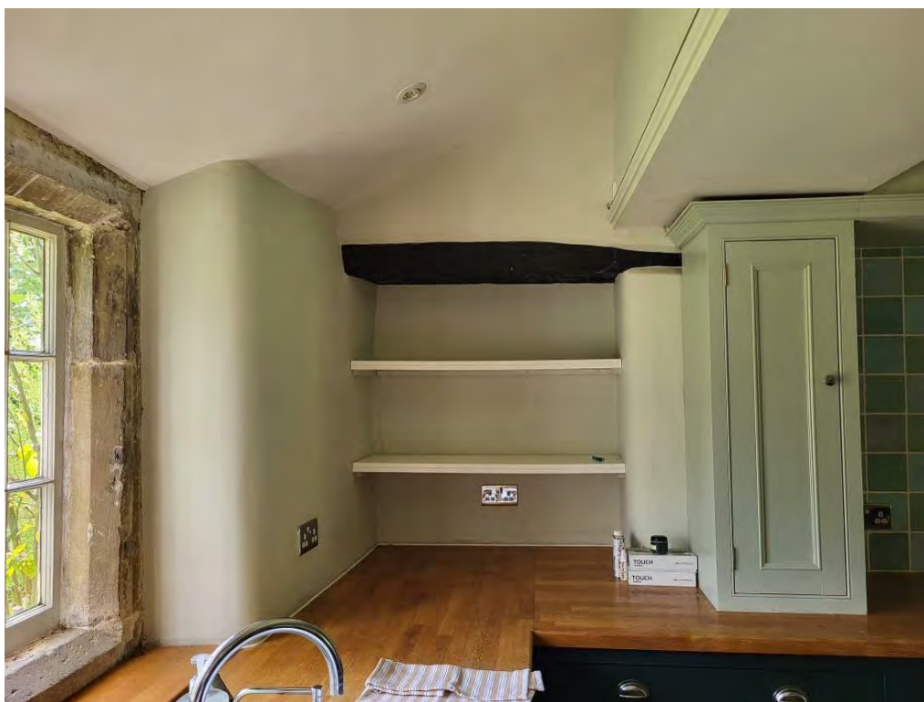
Plate 19: G2, looking south towards recess to left of chimneybreast
