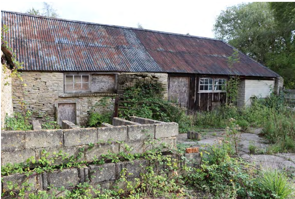
Plate 75: Barn 4: western elevation to courtyard
