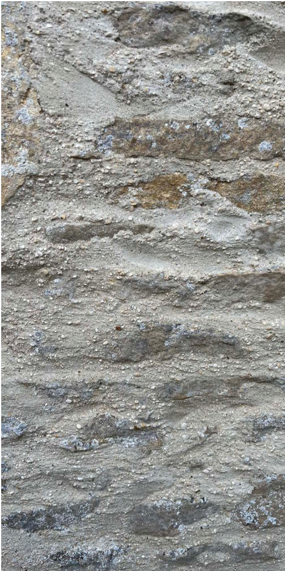
Detail of existing cementitious mortar
