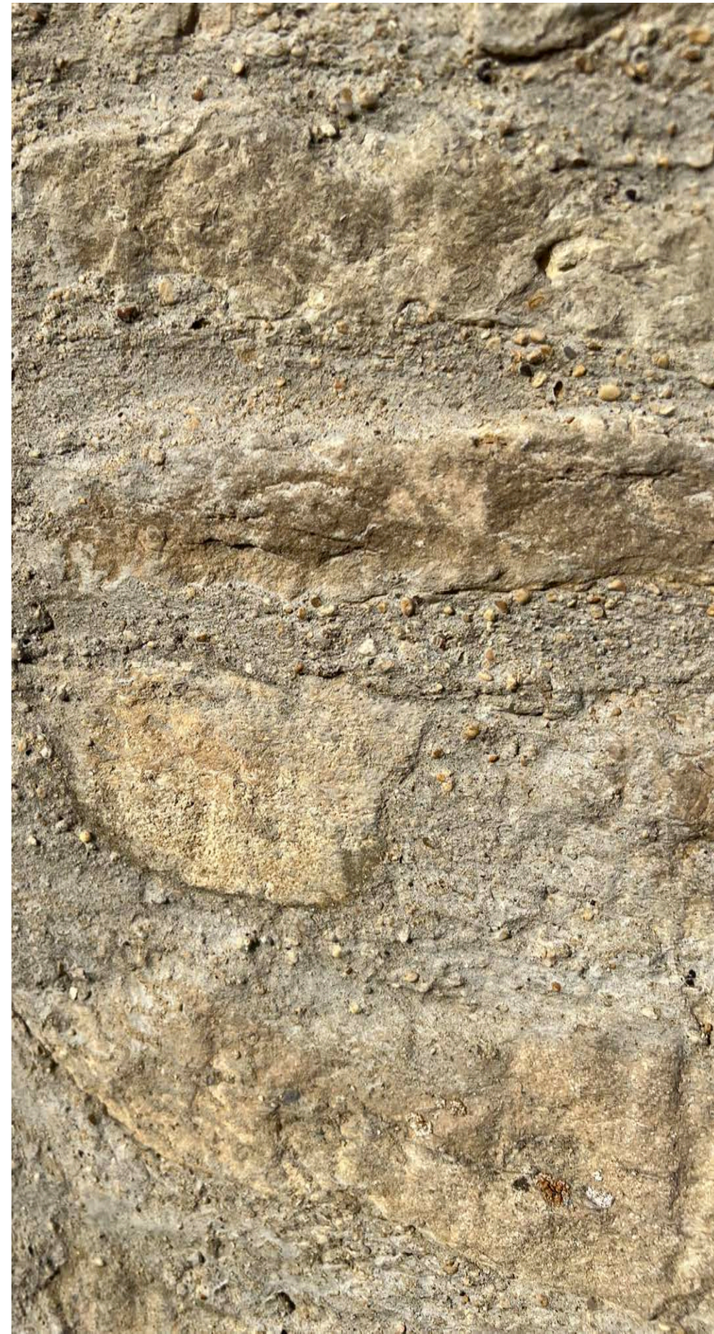
Detail of existing cementitious mortar
