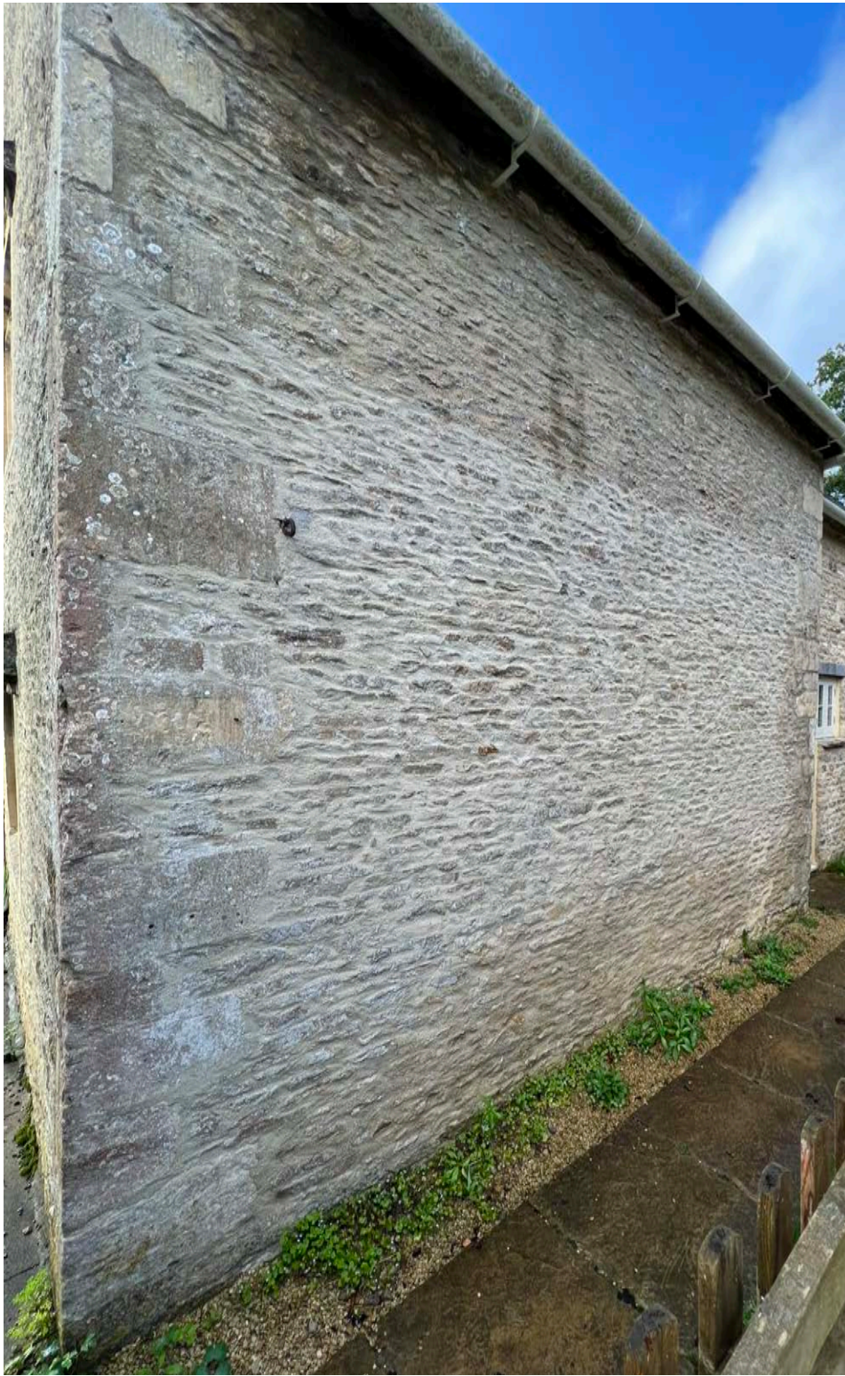
North East Elevation - Showing existing cement mortar
