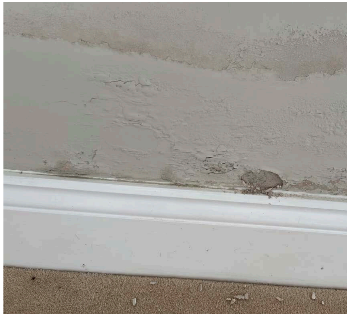
Detail of drawing room damp
