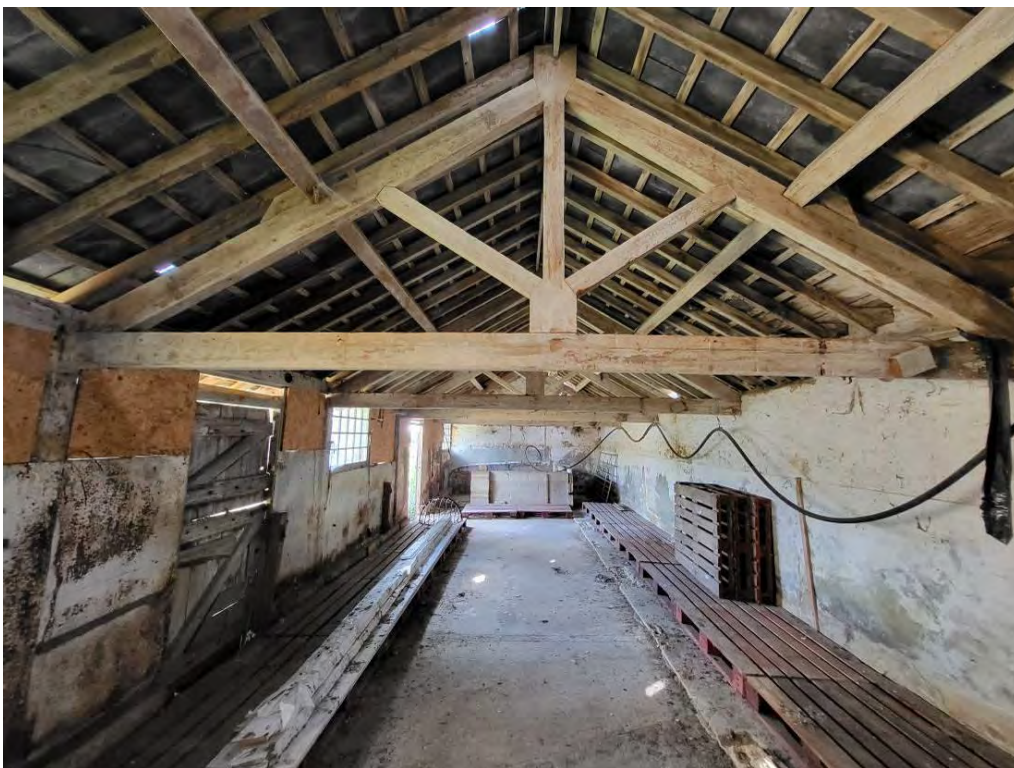
Plate 84: Barn 5, looking south
