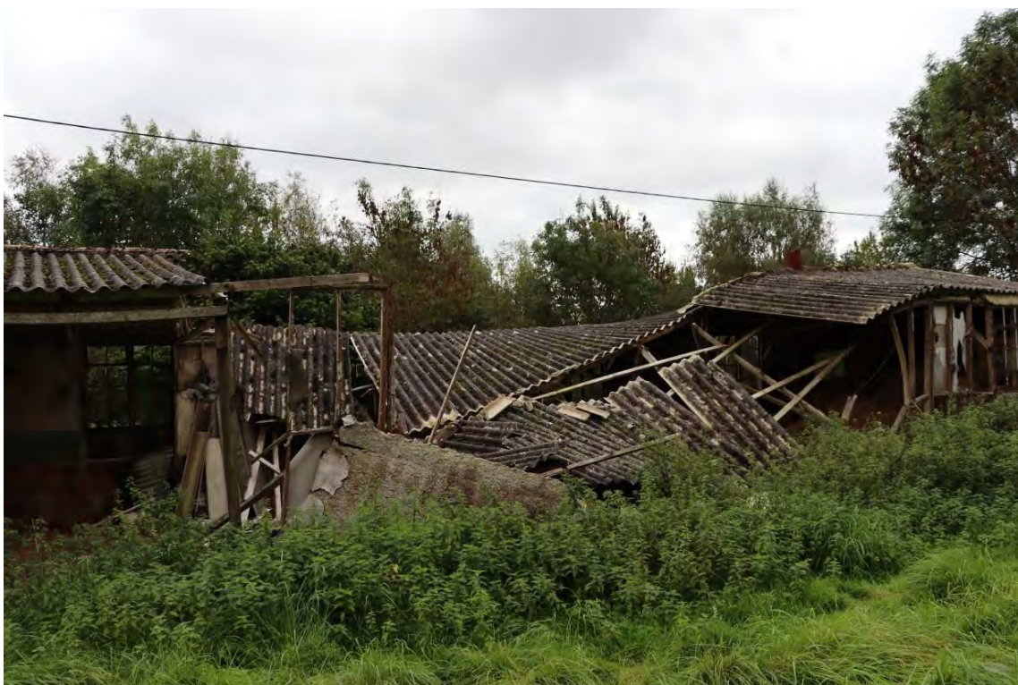
Plate 88: Barn 9: northern range (west elevation)
