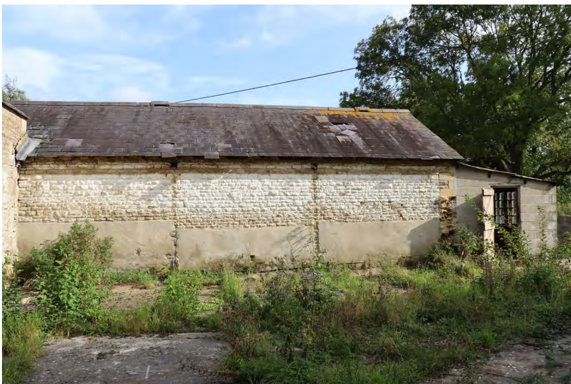
Plate 82: Barn 5: west elevation
