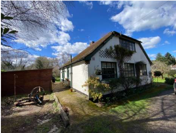
Figure 3. Westerly perspective showing residential property to be demolished under proposed scope of works.
