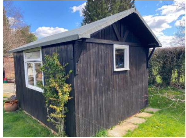
Figure 14. Southern perspective showing garden shed 2 in good state of repair.
