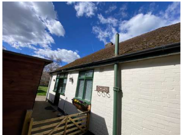
Figure 4. North-westerly perspective showing residential property to be demolished under proposed scope of works.
