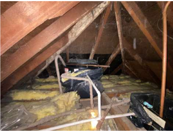
Figure 9. Image showing internal loft space in good state of repair in highest peak of roof.
