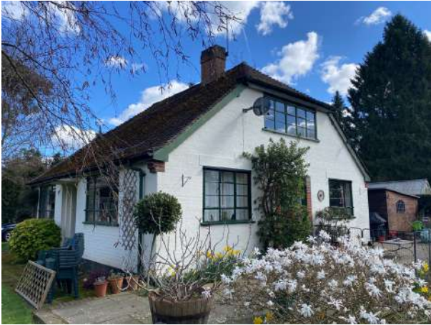
Figure 1. Eastern perspective showing residential property to be demolished under proposed scope of works.
