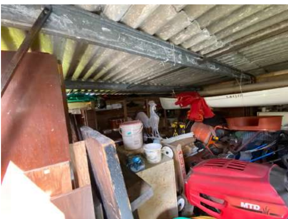
Figure 17. North-eastern perspective showing standalone garage building internal roof space.
