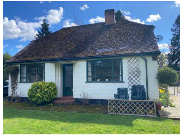
Figure 2. South-easterly perspective showing residential property to be demolished under proposed scope of works. Note brick build construction & well fitted concrete tiles.
