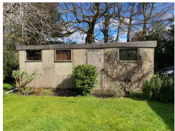
Figure 16. North-eastern perspective showing standalone garage building in good state of repair.
