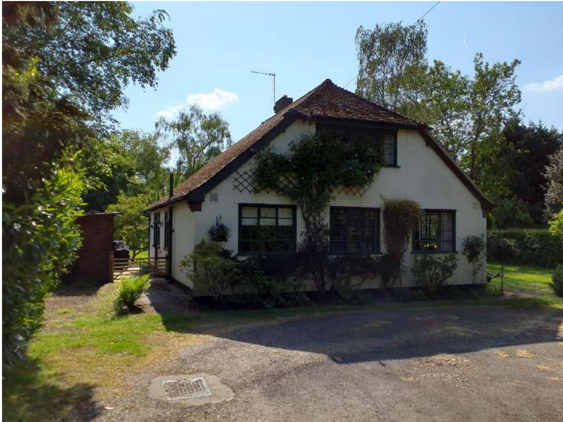
Figure 5 – Looking south west at the existing property.
