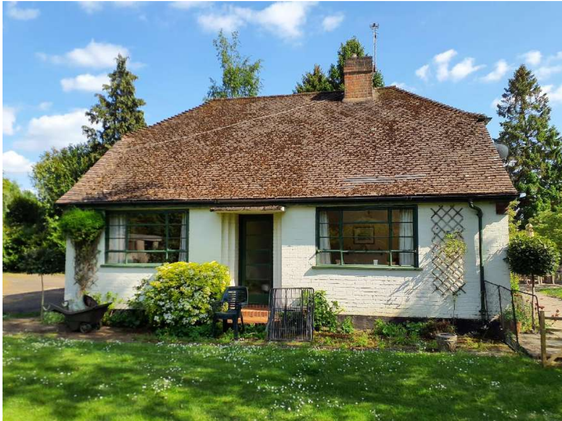
Figure 2 – Looking south east towards the existing dwelling.
