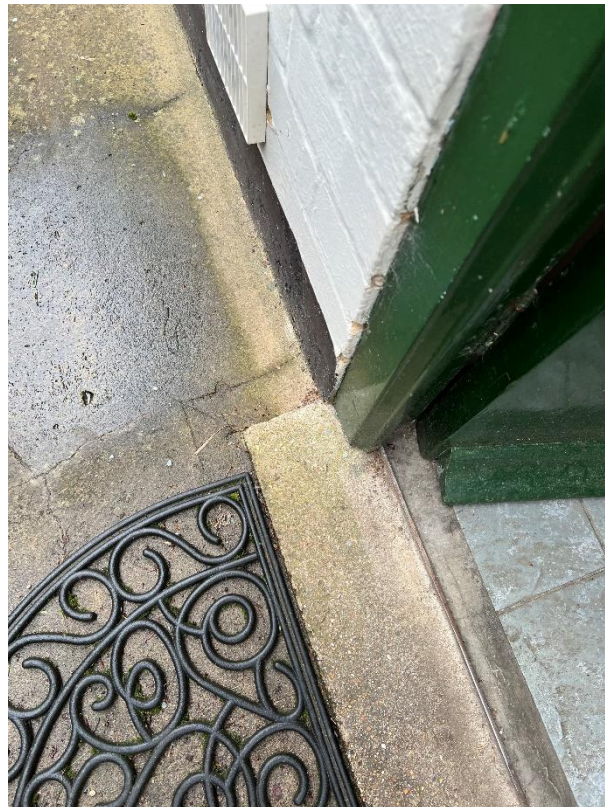
24 – LEVEL THRESHOLD NO D.P.C.
