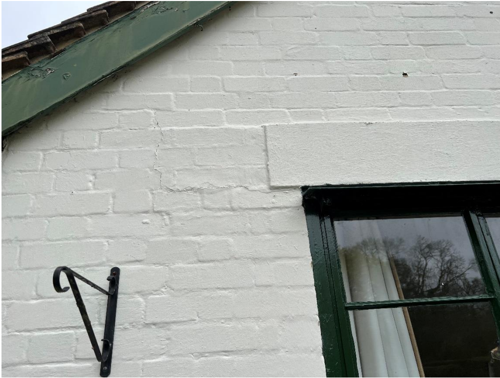
13 – WALL CRACKING
