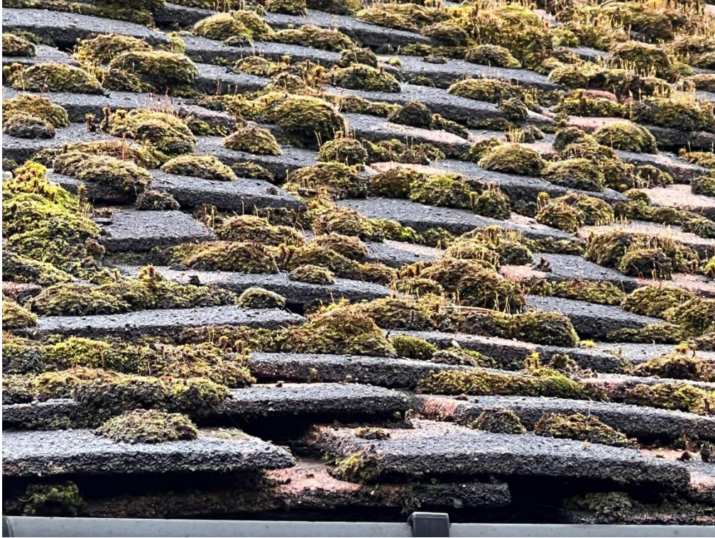
7 – BROKEN/ERODED TILES
