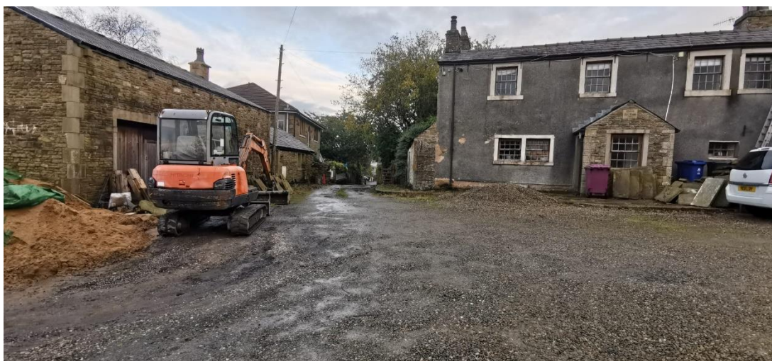
Figure 9: View of access to Hapton Hall Farm looking east, Nov 2023
