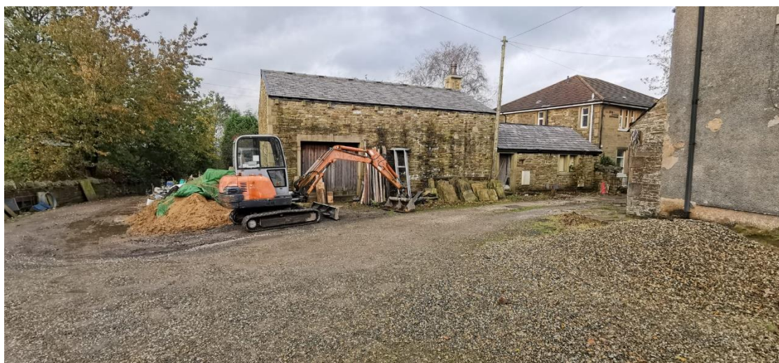
Figure 4: Garage and workshop on site, Nov 2023
