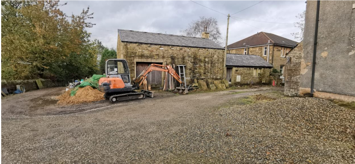
Figure 4: Garage and workshop on site, Nov 2023
