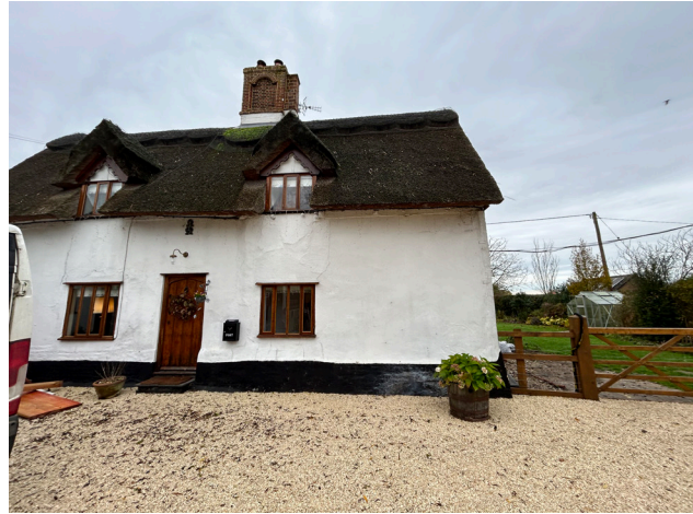
▲ View of the front elevation which is to be affected by the render works.
