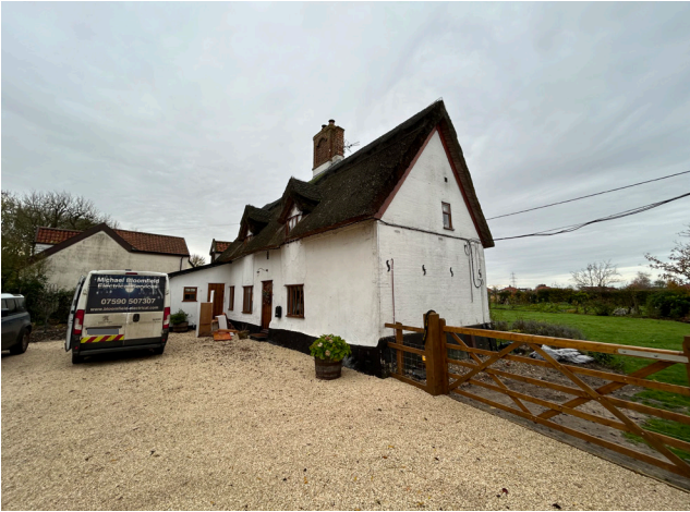
▲ View of the front elevation.
