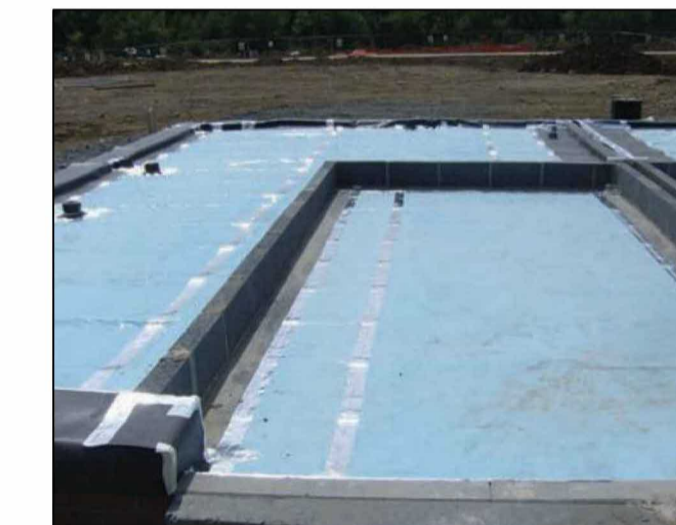
Example of perimeter gas resistant DPM being installed
