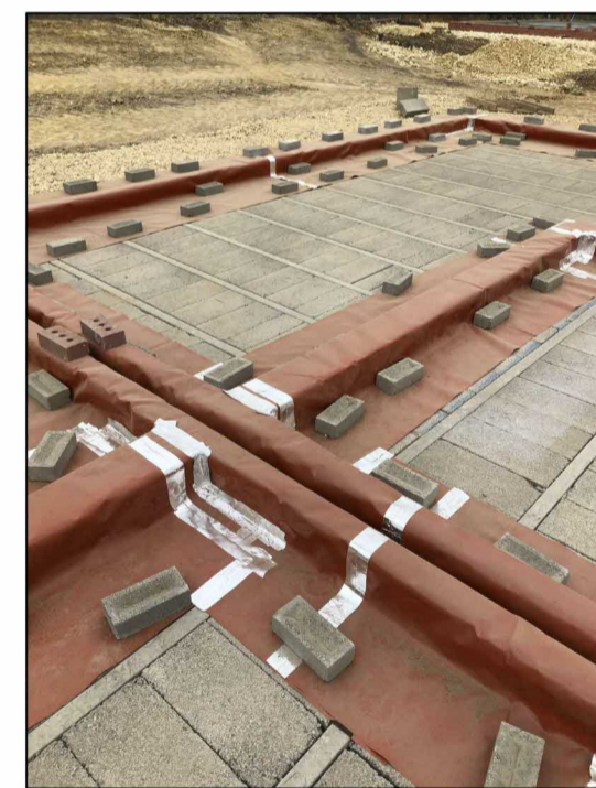
Example of good party wall detailing prior to floor membrane installation
