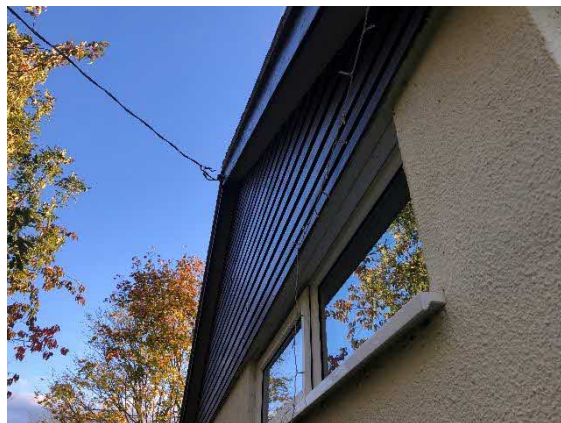
Well-sealed soffits and fascias.
