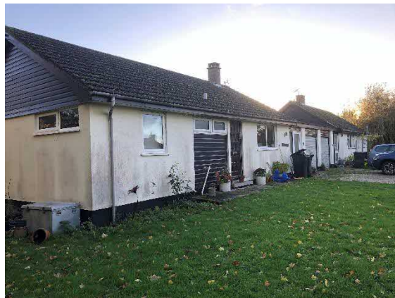
Existing dwellings to be demolished.
