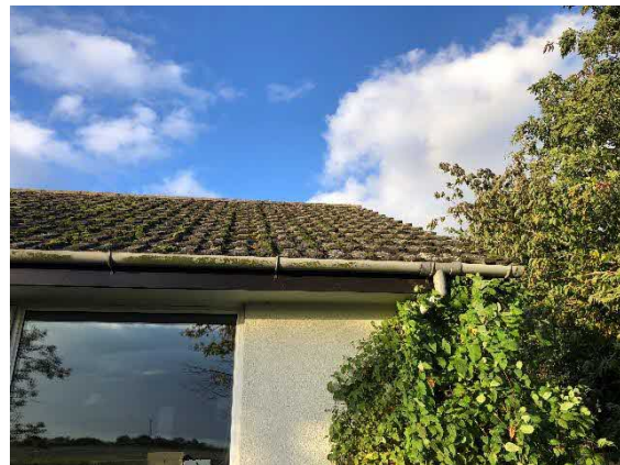
Roof tiles with no lifting or damage.
