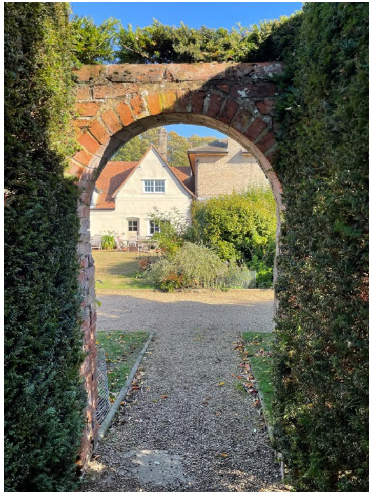
View of side of Holton Hall to North of outbuildings
