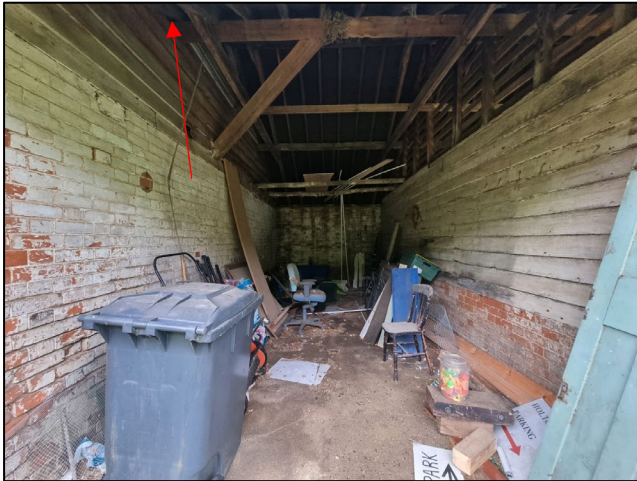
a) Common pipistrelle roost entry point in open bay.
