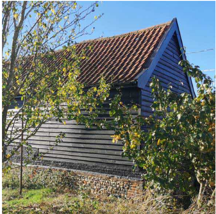
photo showing the existing materials
