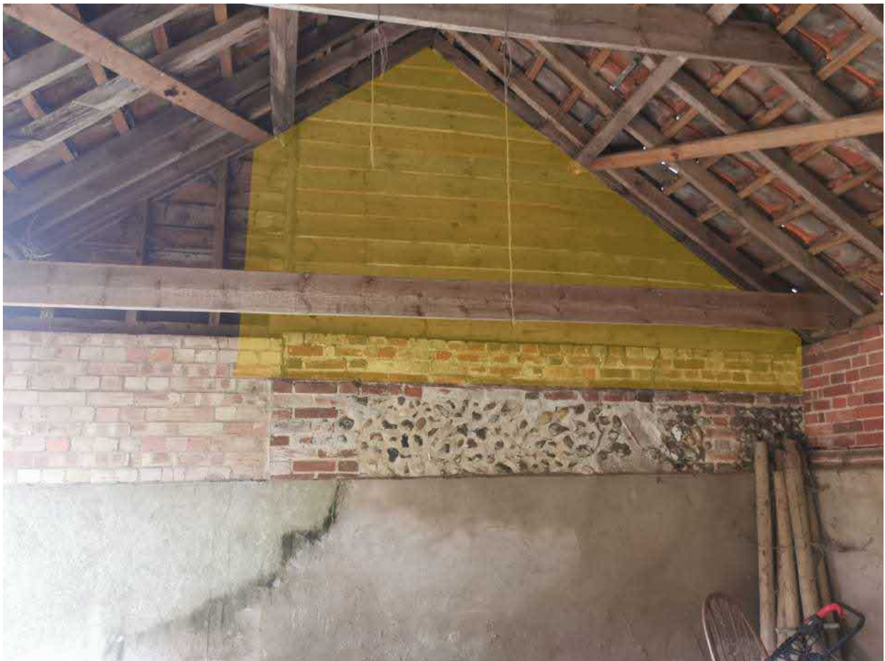
photo showing the area to be insulated in yellow
