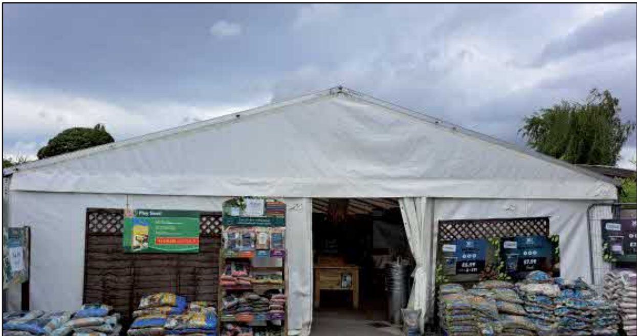
Fig. 3. Existing temporary garden centre shop to be removed.
