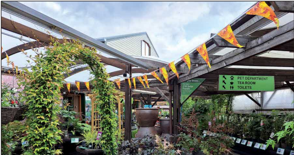
Fig. 4 Existing covered walkways to be removed.
