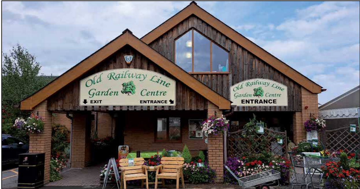
Fig. 5. Existing entrance lobby to be removed.
