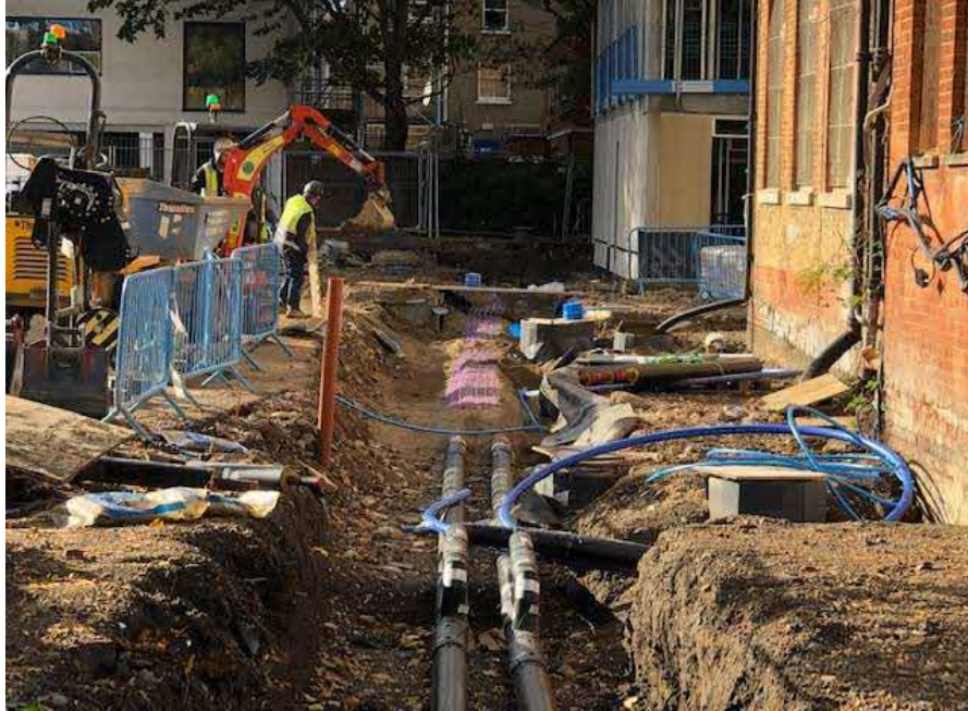
Photographs showing new pipe installations in oversized excavations
