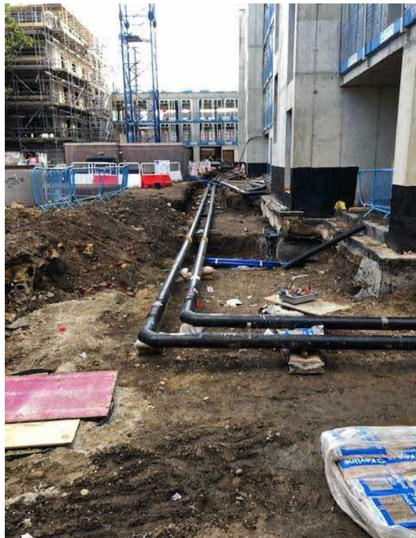
Photographs showing new pipe installations in oversized excavations
