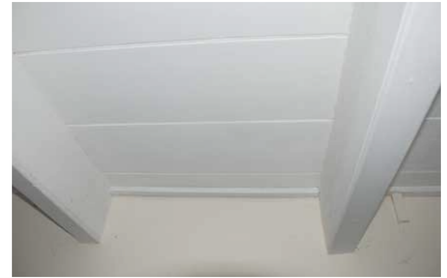
LIVING ROOM CEILING
