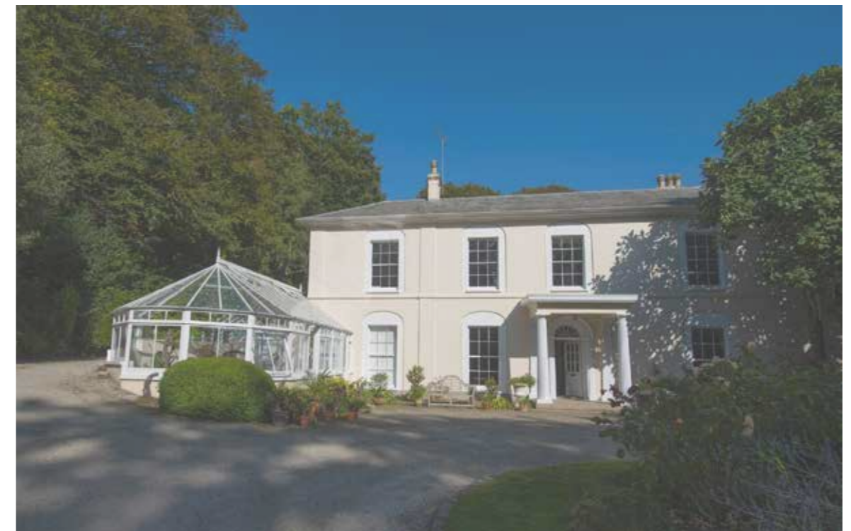
WEST (FRONT) ELEVATION OF TULLIMAAR HOUSE - 2014
