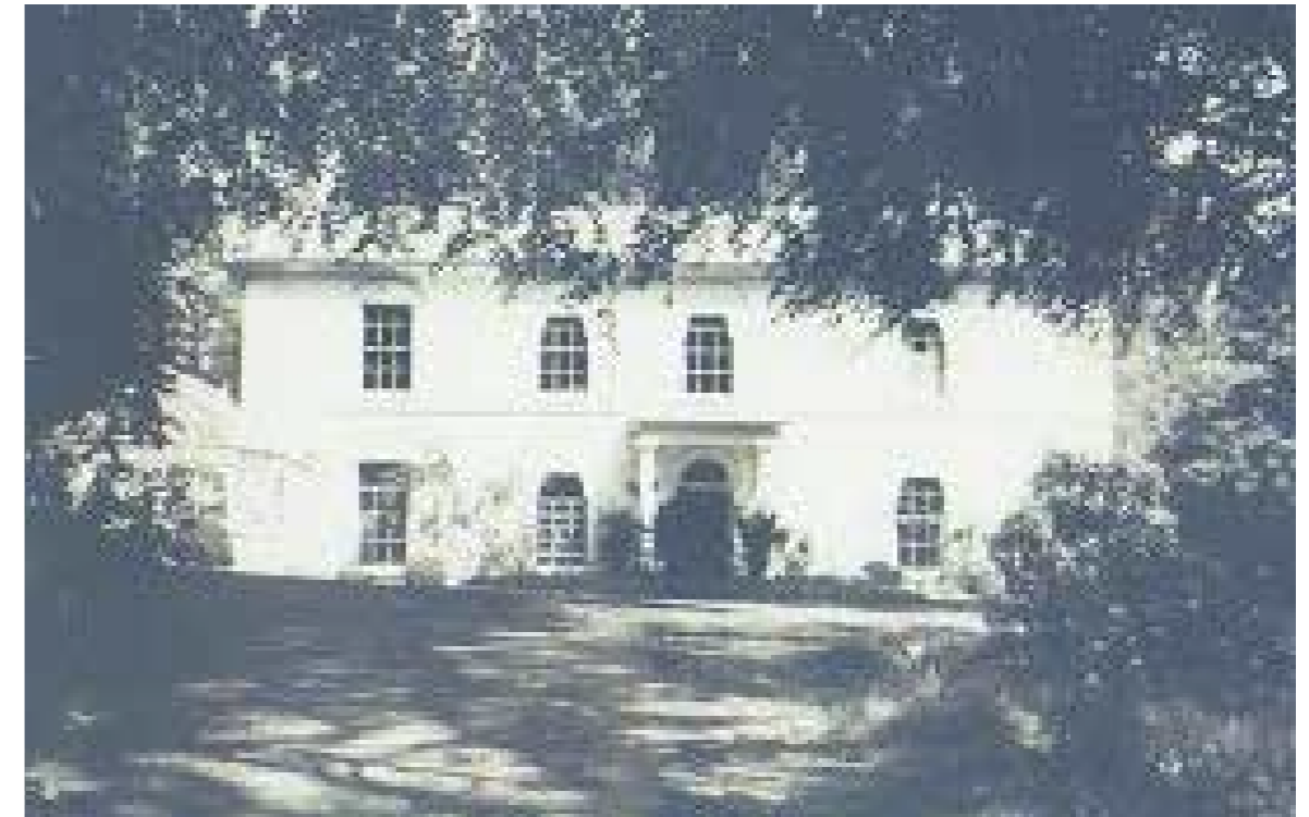
HISTORIC PHOTO OF WEST (FRONT) ELEVATION OF TULLIMAAR HOUSE - DATE UNKNOWN
