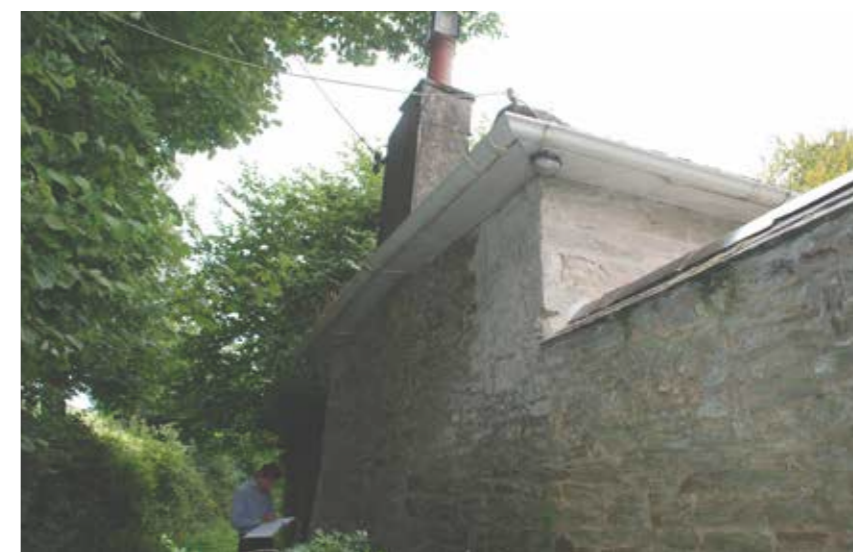
VIEW OF GARDENER'S COTTAGE PART NORTH ELEVATION
