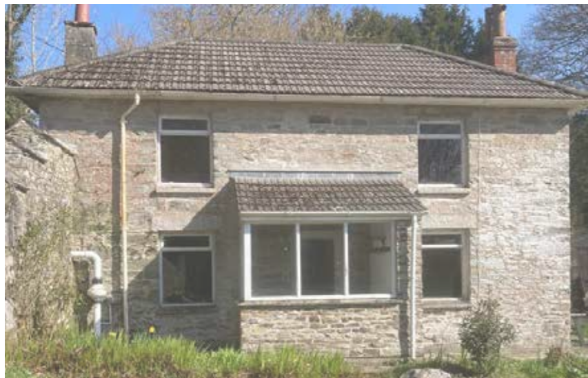
VIEW OF GARDENER'S COTTAGE WEST ELEVATION
