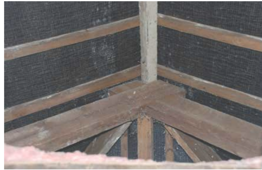
INTERNAL VIEW OF ROOF STRUCTURE
