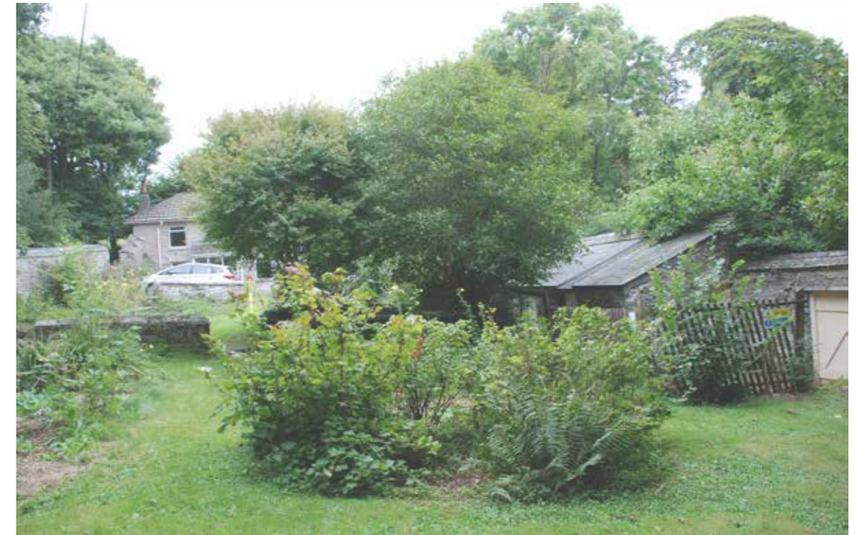
VIEW OF GARDENER'S COTTAGE & STOVE HOUSE FROM THE VEGETABLE GARDEN TO THE WEST
