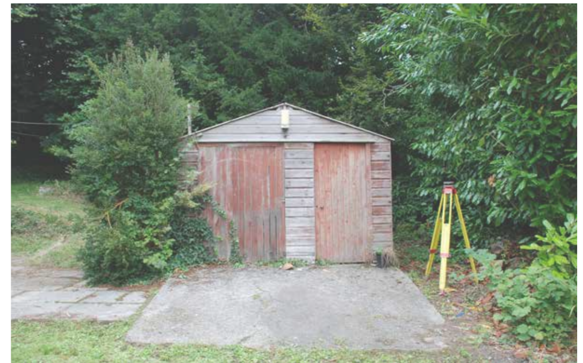
VIEW OF THE EXISTING TIMBER GARAGE TO SOUTH EAST OF THE GARDENER'S COTTAGE
