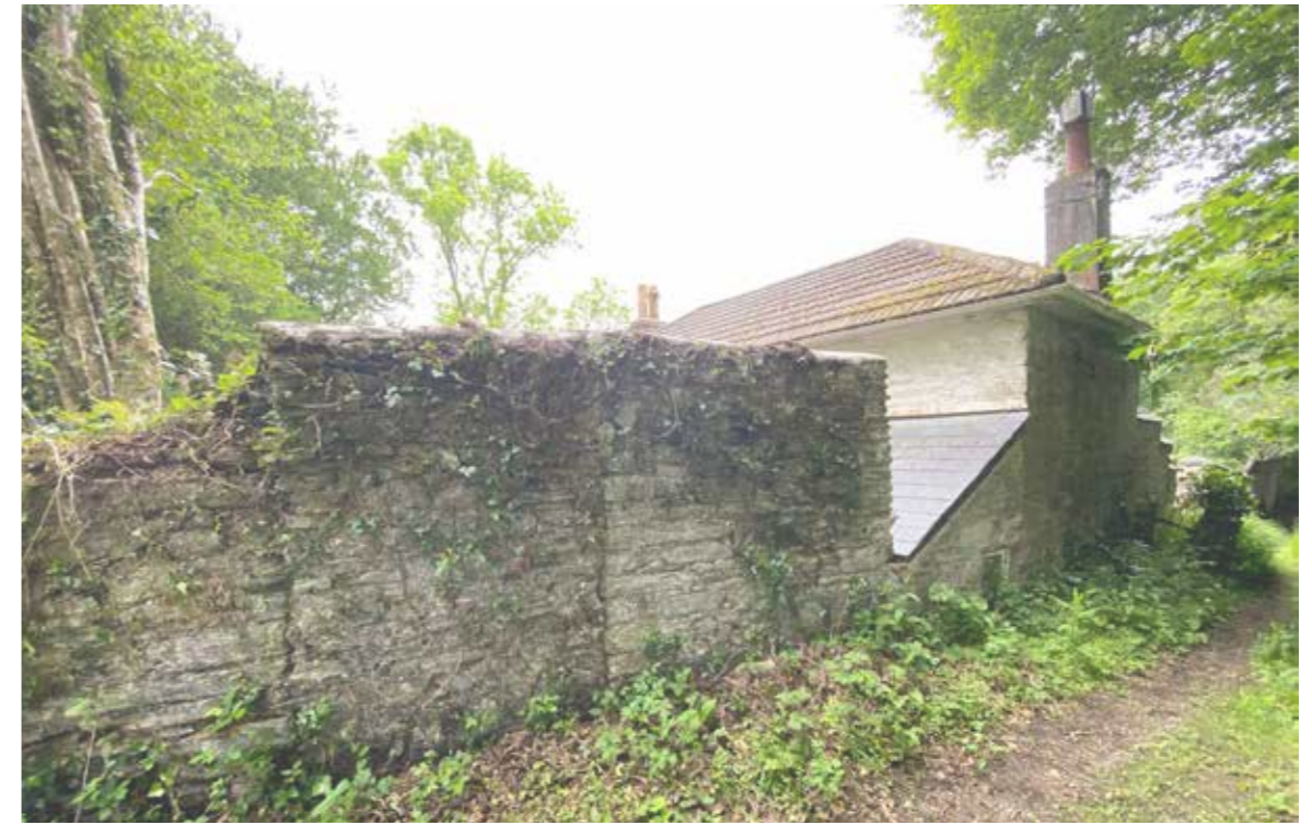
VIEW OF GARDENER'S COTTAGE PART NORTH ELEVATION AND ADJOINING BOUNDARY WALL
