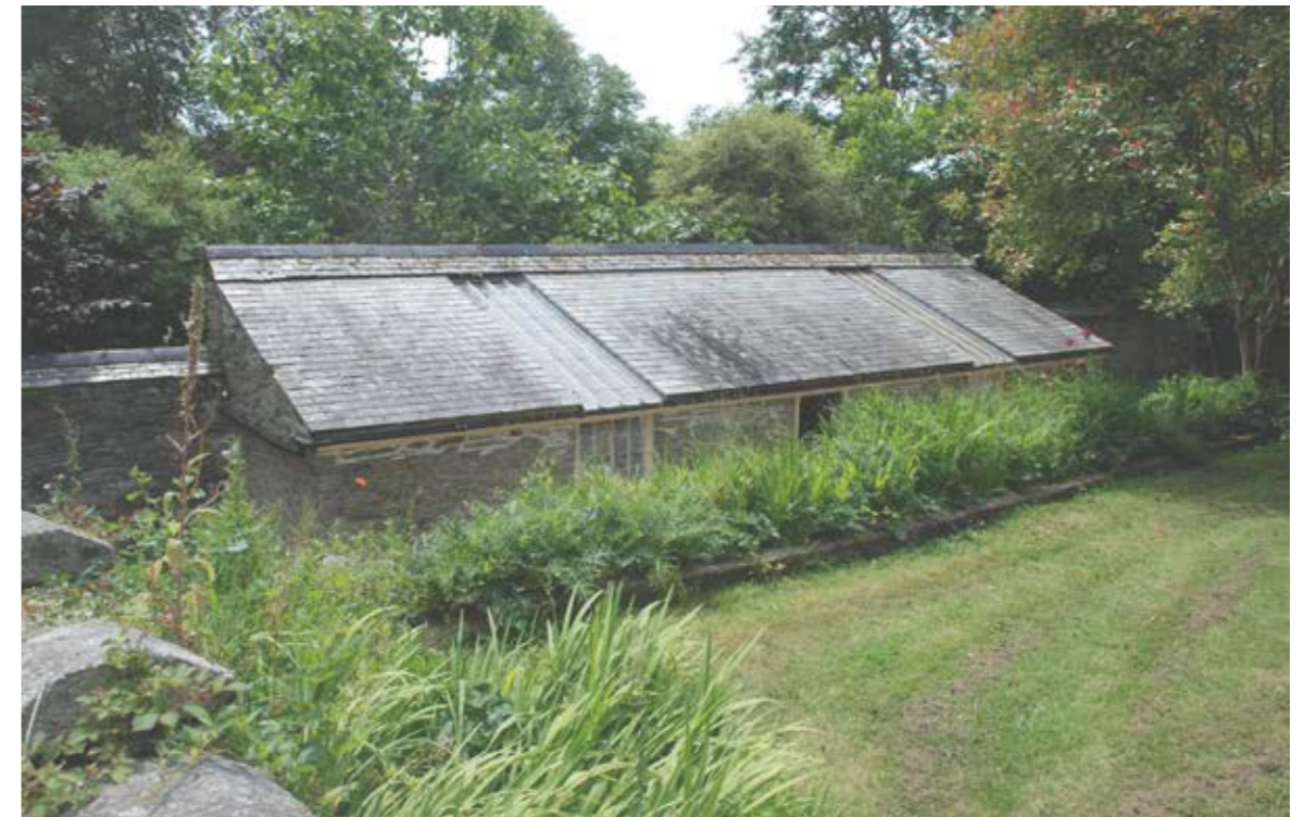
VIEW OF STOVE HOUSE FROM GARDENER'S COTTAGE
