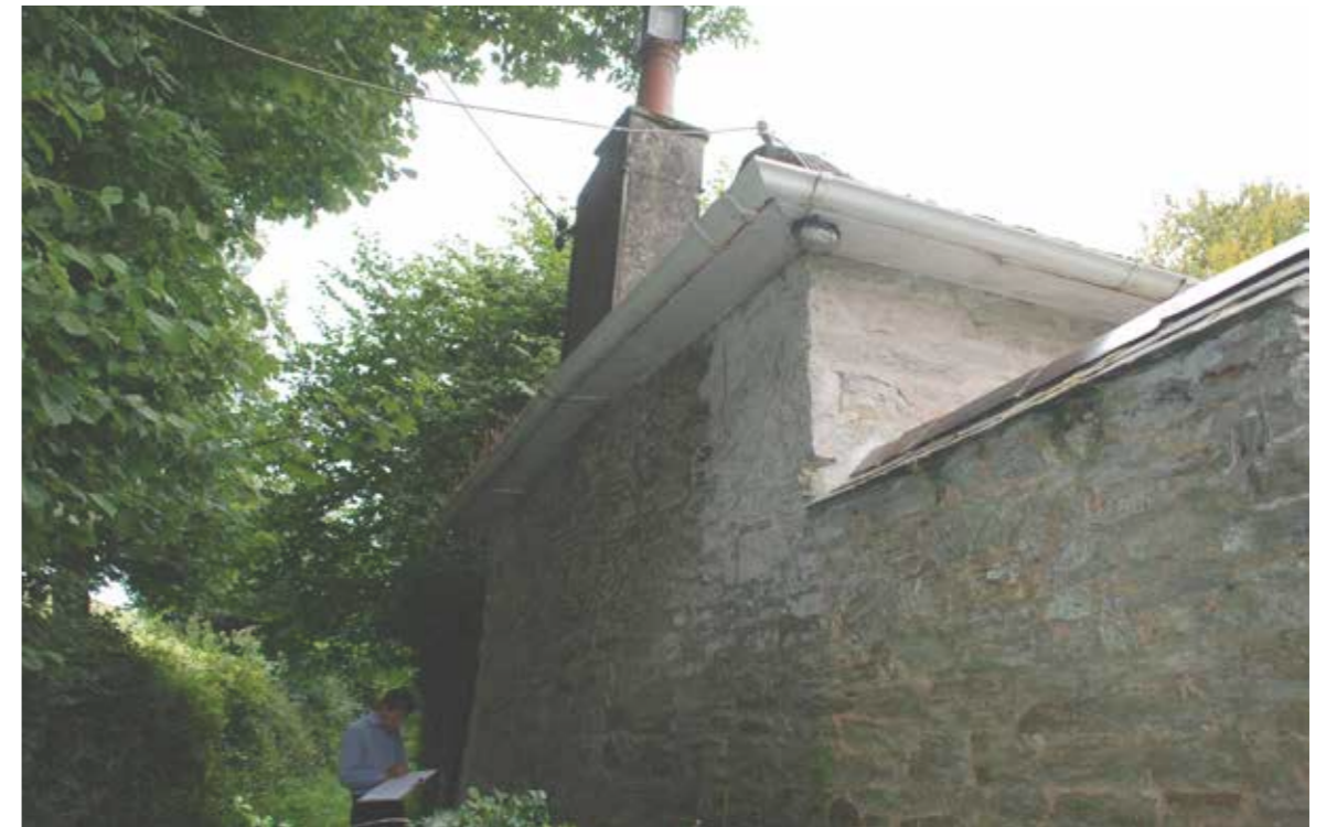
VIEW OF GARDENER'S COTTAGE PART NORTH ELEVATION
