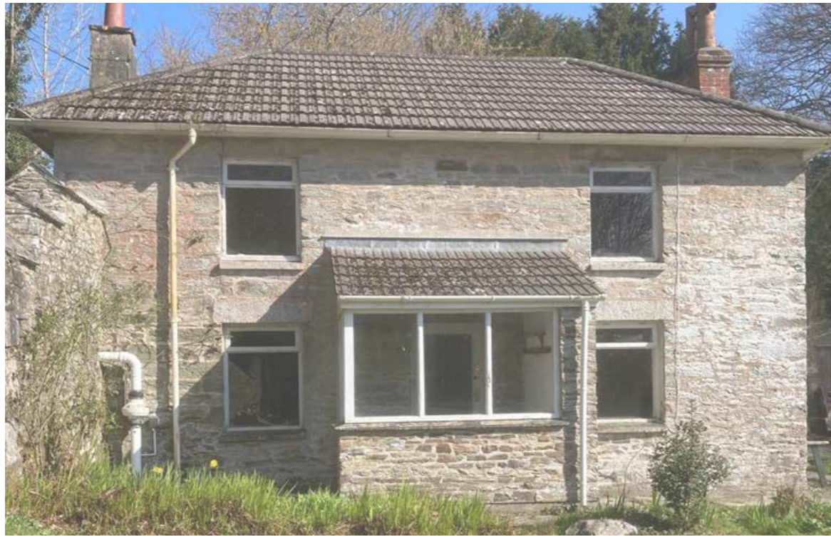
VIEW OF GARDENER'S COTTAGE WEST ELEVATION
