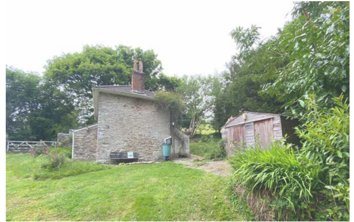
VIEW OF GARDENER'S COTTAGE SOUTH ELEVATION WITH TIMBER GARAGE TO SOUTH EAST
