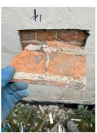
Showing detail of mortar and brick face adhering to cement render plus damp spores beneath the render, iron nail embedded in cement mortar
