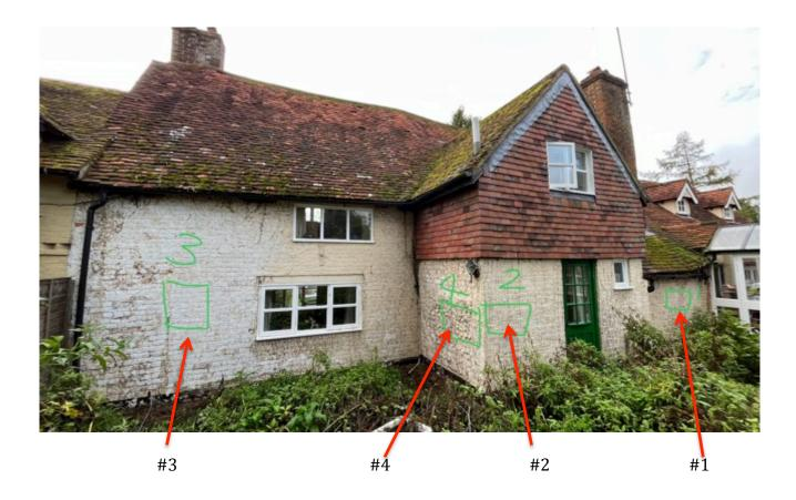
All test panels subjected to 2no. applications of Paint-Rid<sup>™</sup> – first coat left over night, second coat left for a few hours dwell time.
